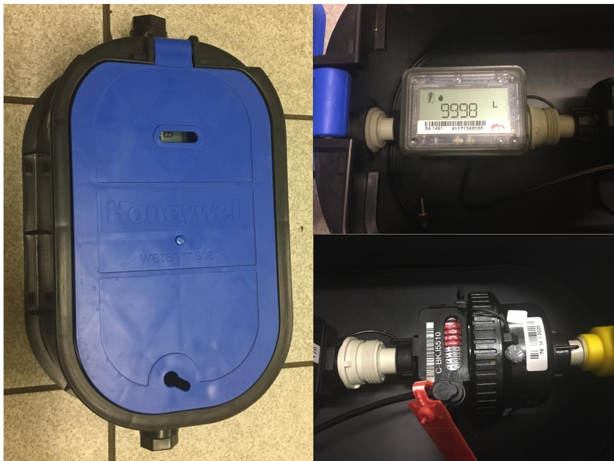
Image 4.1 Water meter with water management device (top) and meter (bottom). Source: Author.
