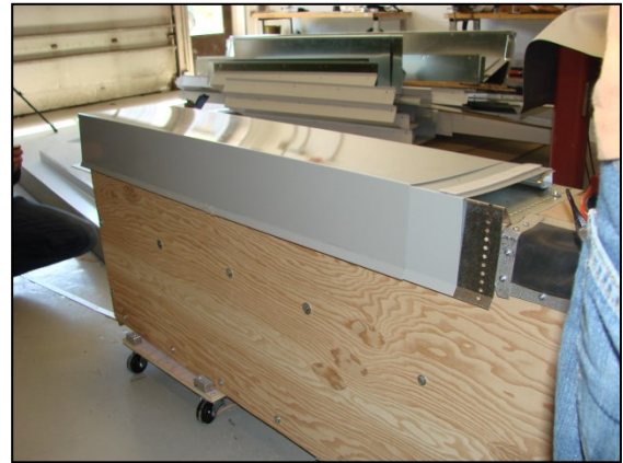
(b) Clipping the coping on anchor clips
