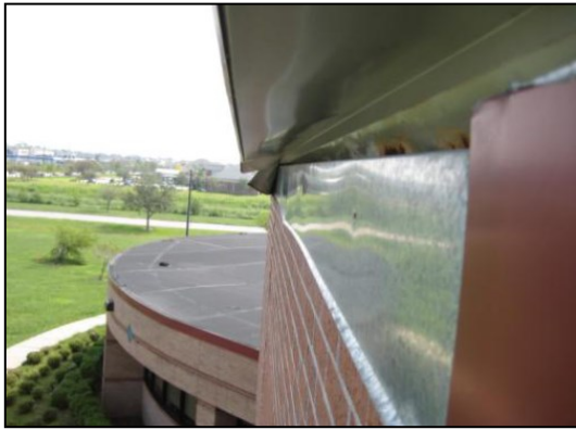
(a) Flashing disengaged from cleat
