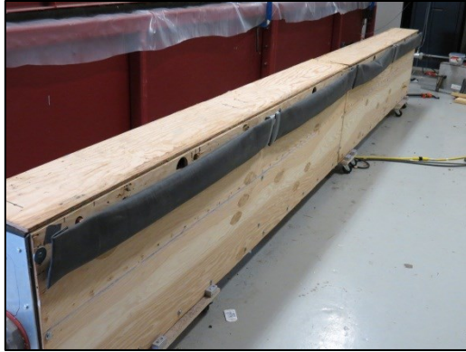
(g) Pressure bags installed along entire edge length
