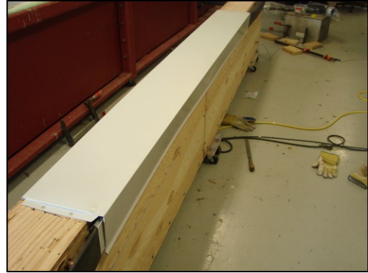
(h) Installation of coping
