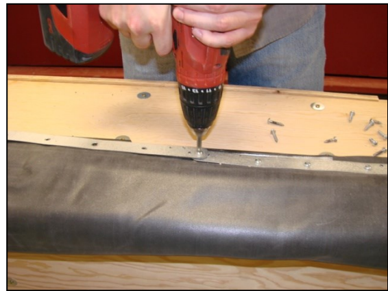
(b) Cleat installed
