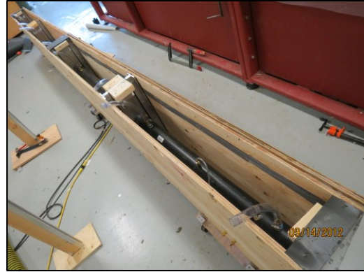
(b) Installation of edge substrate
