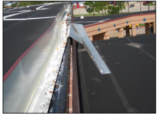
(b) Cleat came off the edge substrate
