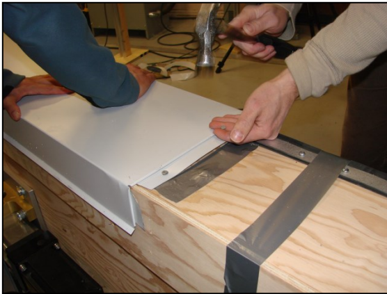
(a) Hooking the coping on the cleat
