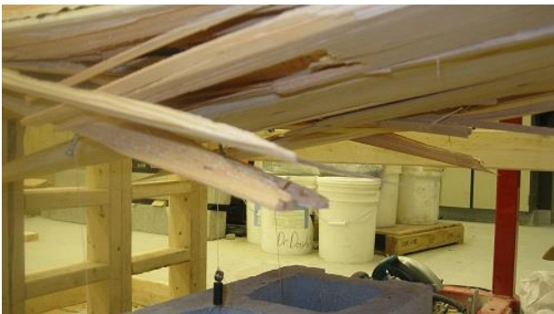
Simple Span 5 Board Failure
