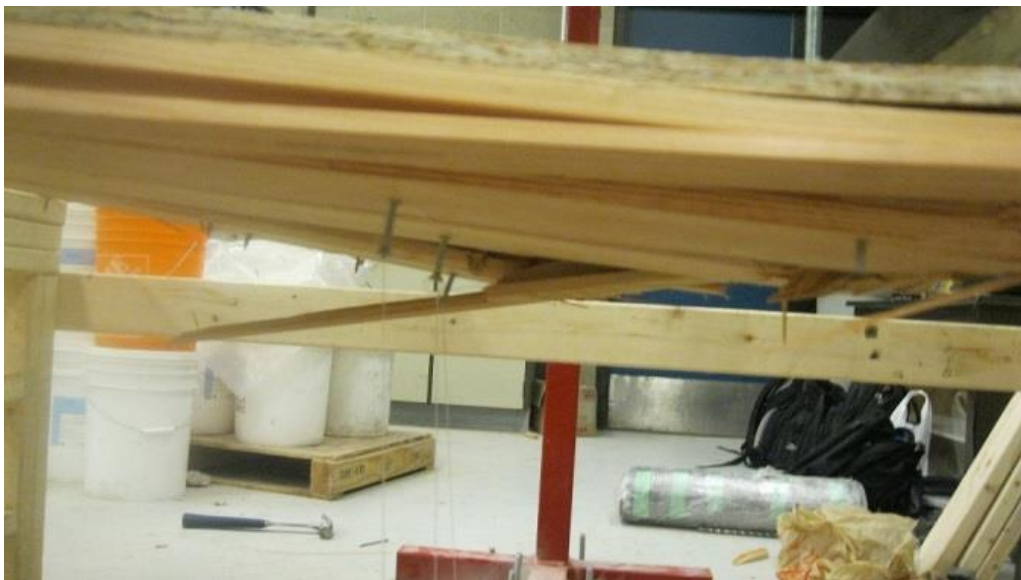
Simple Span 5 Board Failure with Sheathing
