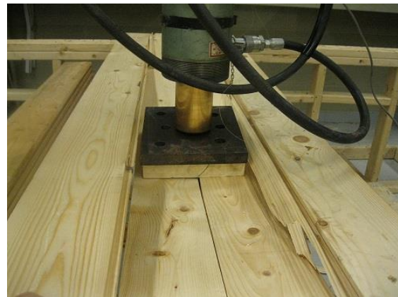
Simple Span 4 Board Failure
