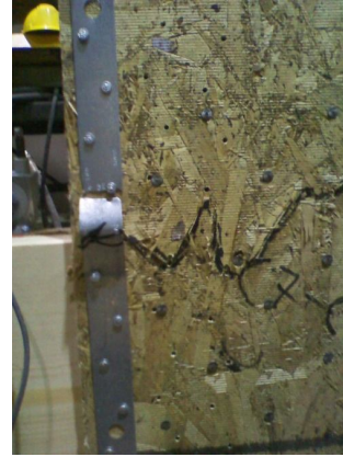
(b) Metal strap and OSB failure right face
