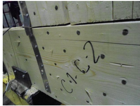
(b) Metal strap failure right face
