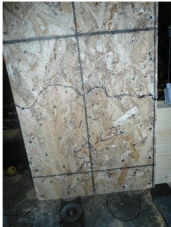
(a) OSB failure left face
