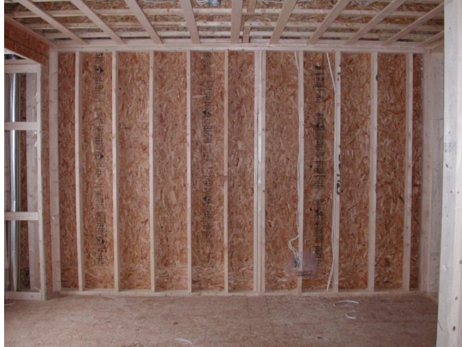
Figure 1.1: Typical light-frame wood shearwall (interior view)
