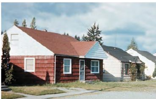
a) Residential house from the 1960's
