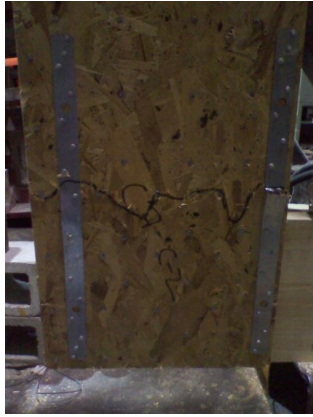
(a) Metal strap and OSB failure left face
