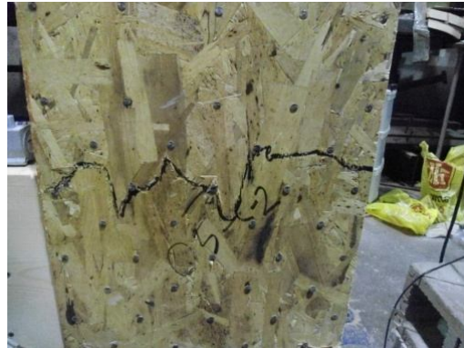
(b) Exterior OSB sheathing failure
