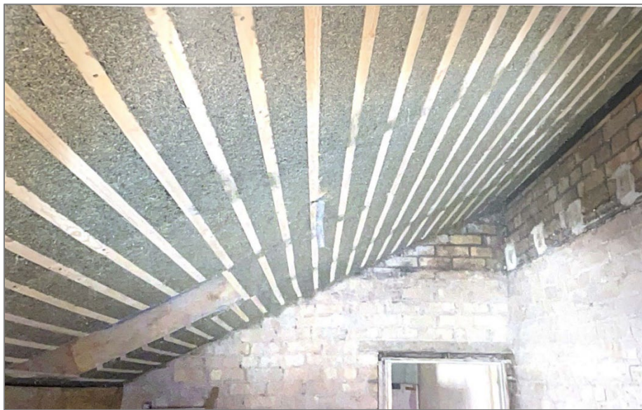
Figure 6- Hempcrete roof application (Stanwix & Sparrow, 2014)
