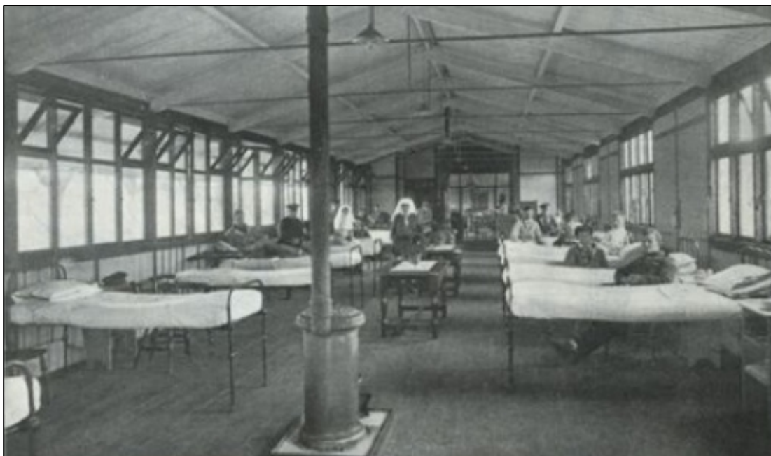
Figure 7: A Permanent Ward of No. 12 Canadian General Hospital. Source: The Bramshott Souvenir Magazine (London: Polsue Ltd., 1918), 22.
