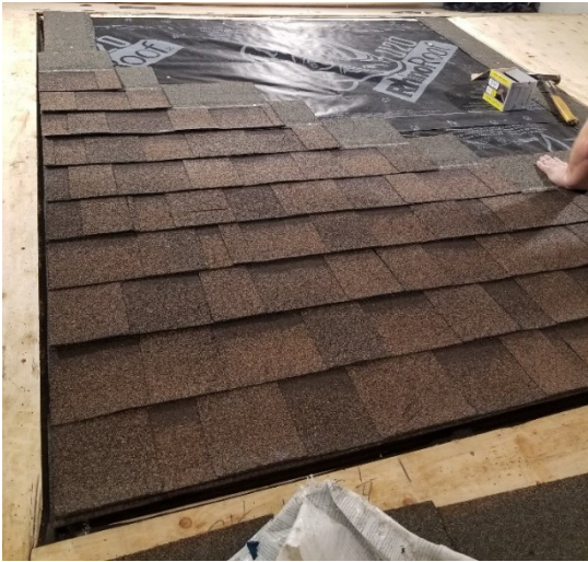
Figure 2. 14 Shingle Installation for mock-up construction at the University of Ottawa
