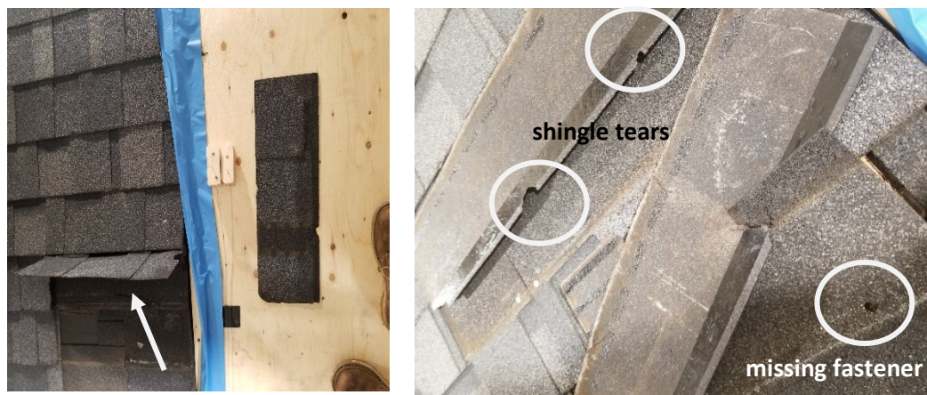
Figure 5.18 Field zone failure mode observed at the end of the test (Failure Mode 1,3,4)
