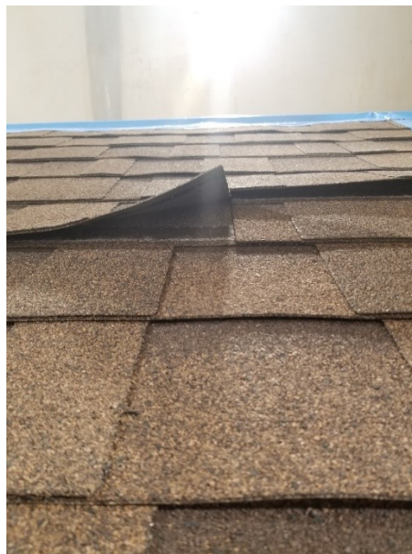
Figure 5.16 Failure mode for the tested “New Edge 2020” mock-up
