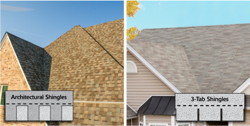
Figure 2. 15 Types of Asphalt Shingles [25]
