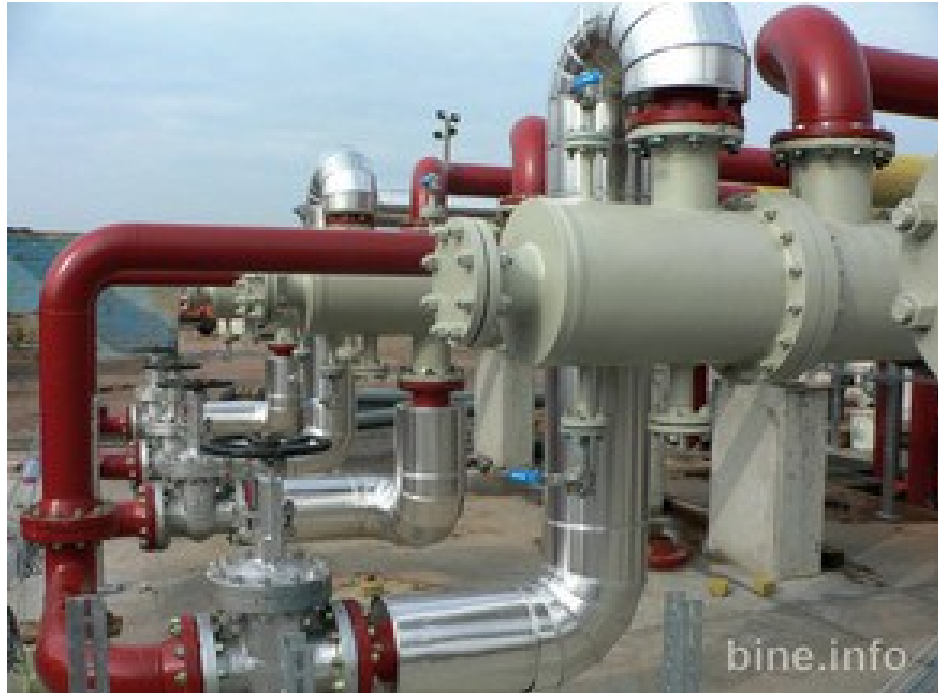
Figure2.1: ORC system of a geothermal power plant [23]
