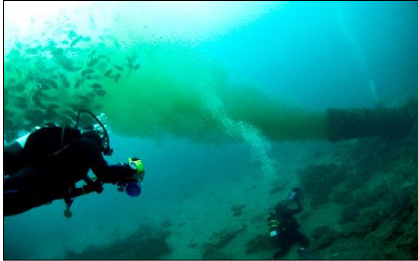
Figure 1-2: Brine discharged of the Delray Beach sewage outfall, Florida, USA, using submerged pipe (Prins, 2016).
