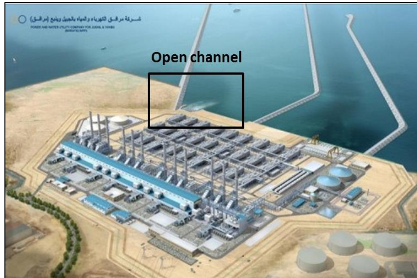
Figure 1-1: Brine discharged directly from Al Jubail desalination plant into the Gulf using an open channel method (surface discharge) (Picow, 2009).
