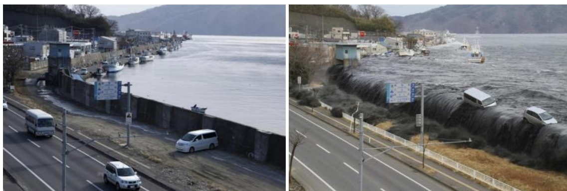
Figure 10: (a) Seawall; and (b) Tsunami overtopping during the 2011 event in Miyako, Japan (Source: Reuters).
