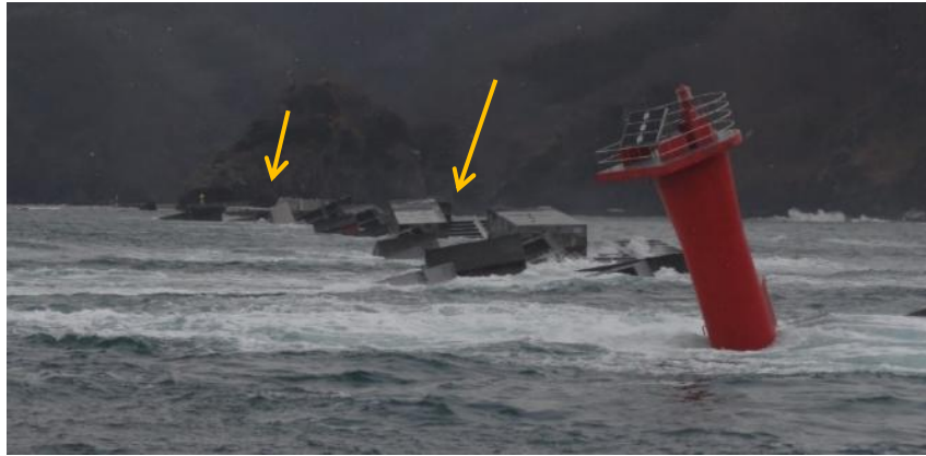
Figure 11: Breakwater damage during tsunami event
