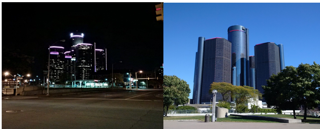
Figure 20 - Le Renaissance Center
