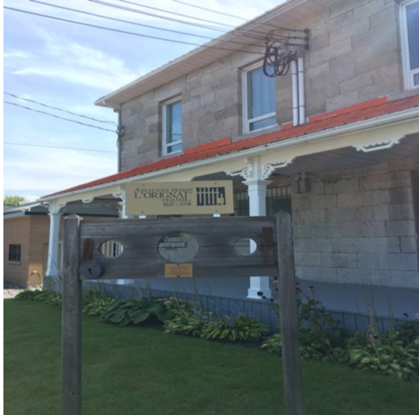
Figure 2: Exterior of L'Original Old Jail
