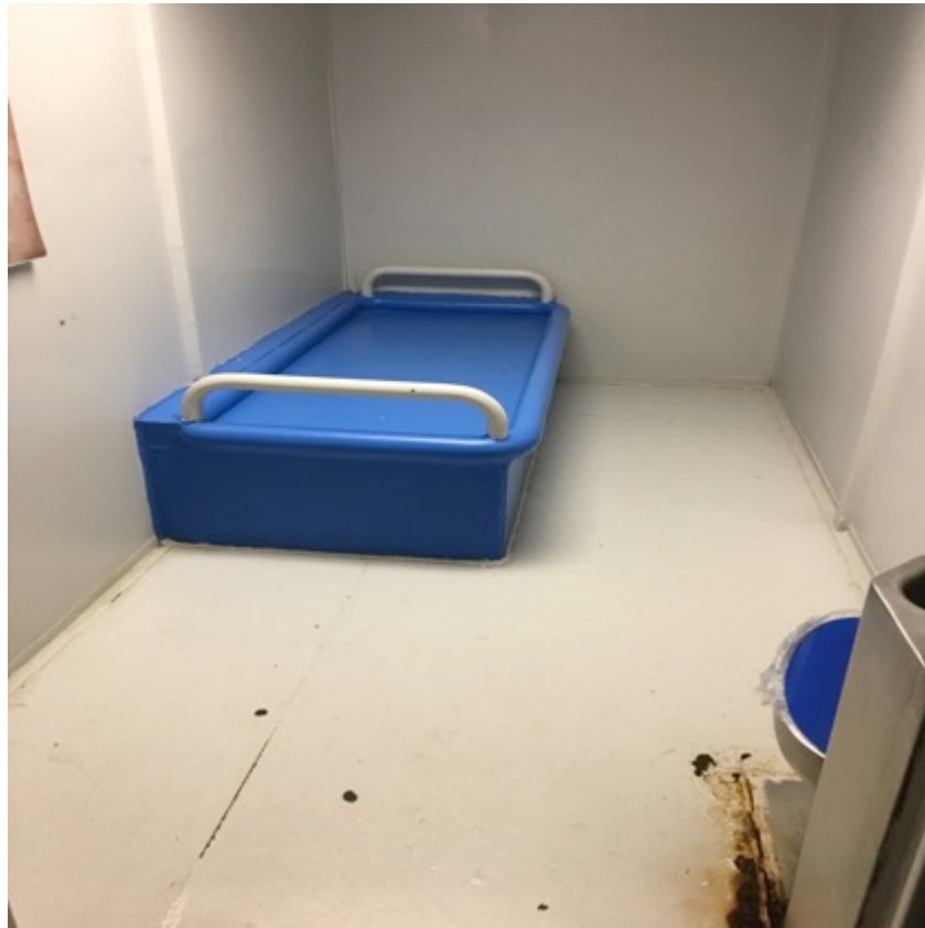
Figure 9: Interior of the solitary confinement cell at L'Orignal Jail
