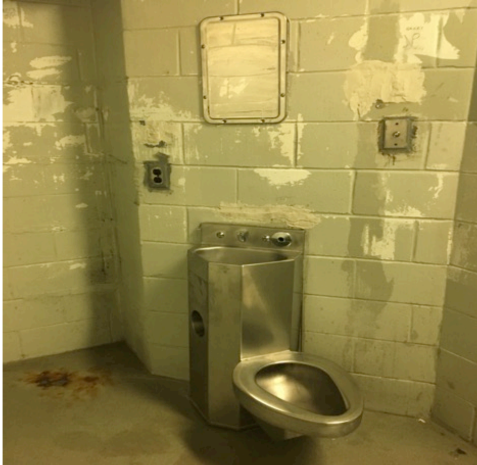
Figure 13: The interior of a long-term segregation cell at Kingston Penitentiary
