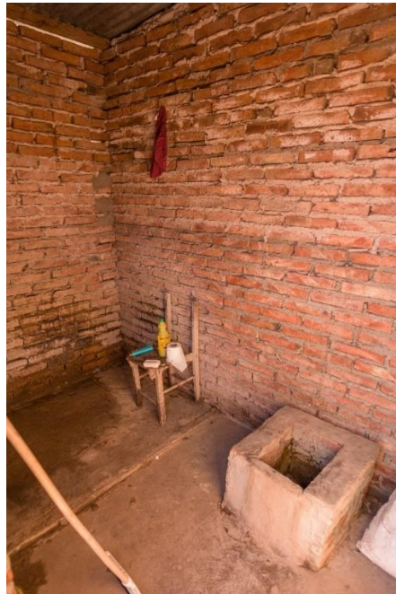
Figure 23: In marginal neighbourhoods, dwellings with poor sanitation are typical. Evacuation is not connected to the sewage network or septic tank. Photo by José Francisco Malina
