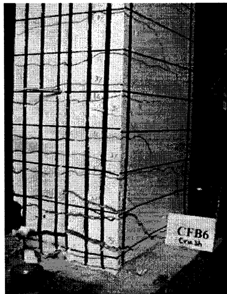
(g) Beam Failure
