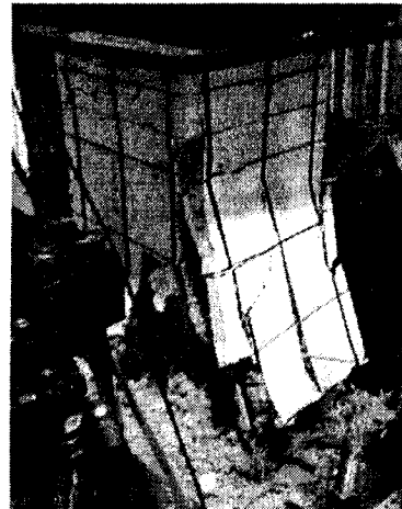
(f) Concrete Crushing
