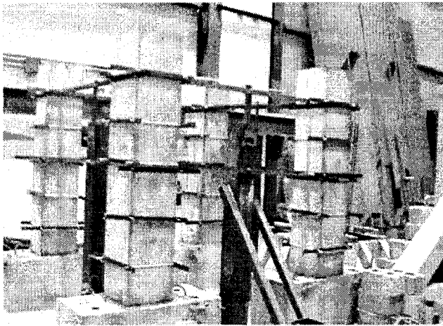
(a) Formwork for Long and Short Columns
