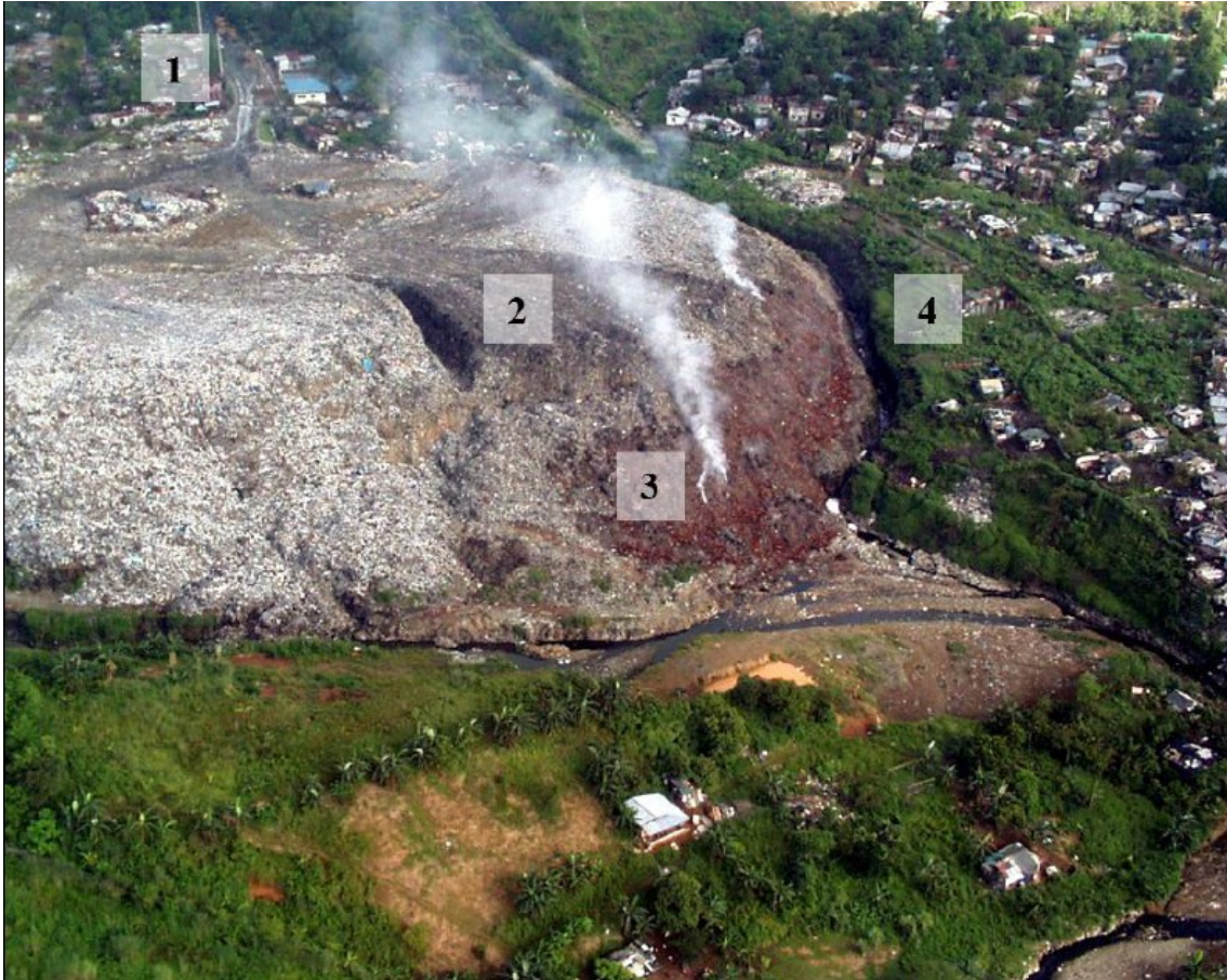
Figure 2-10: Smoke plumes after landfill slope failure in Philippines (Merry et al., 2005).
