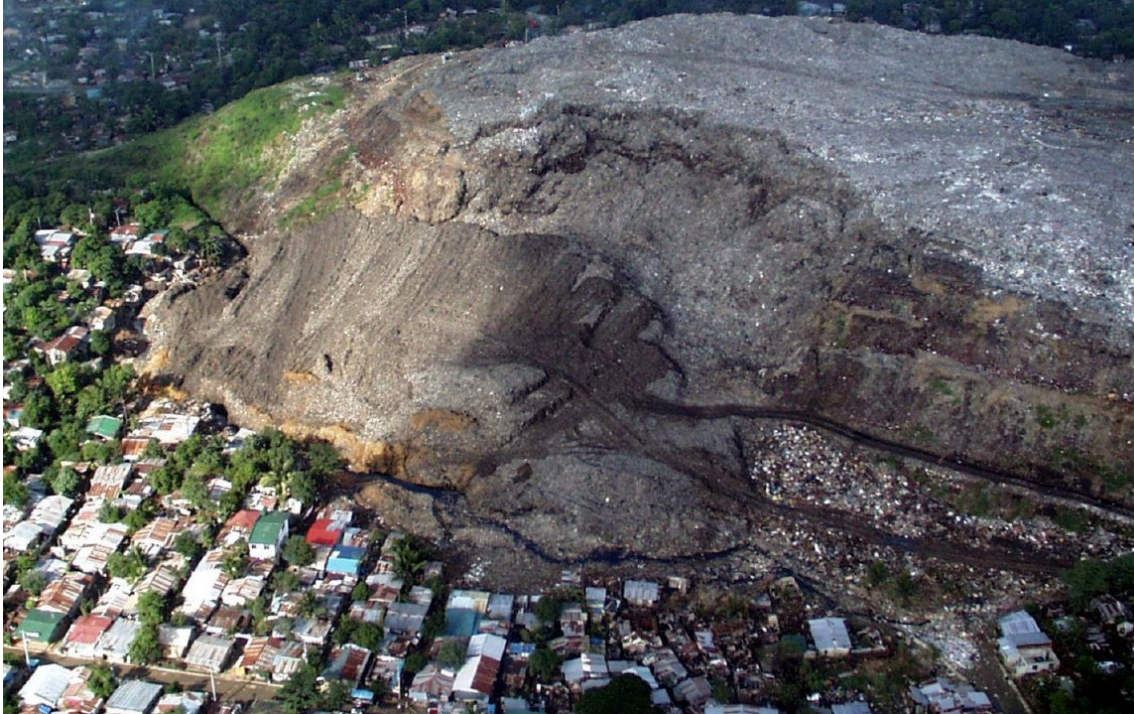
Figure 2-11: Aerial view of 12.7-hectare Payatas landfill, Philippines, with slope failure and homes visible in foreground (photo by S. M. Merry) (Jafari & Stark, 2012; Merry et al., 2005).
