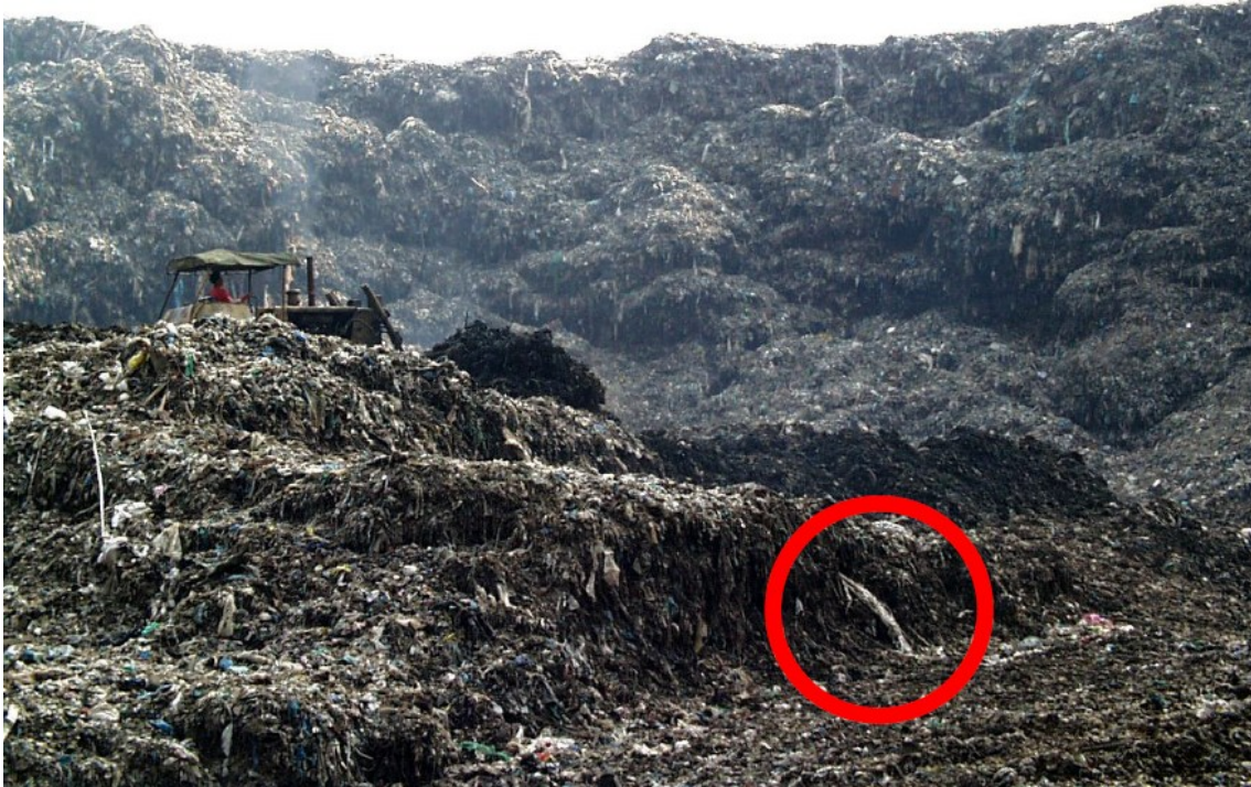
Figure 2-9: Leachate flowing from an exposed MSW landfill (Merry et al., 2005).
