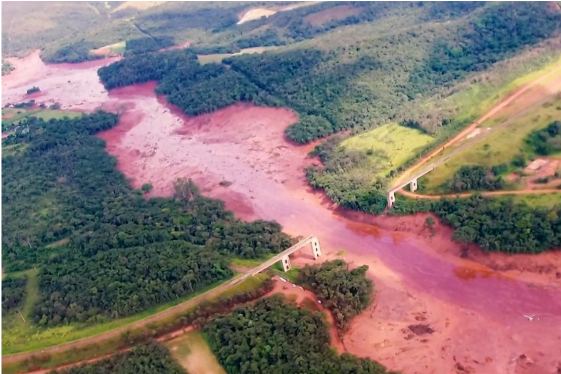
Figure 2-4: Collapse of Córrego do Feijão mine in Brumadinho, Brazil.
