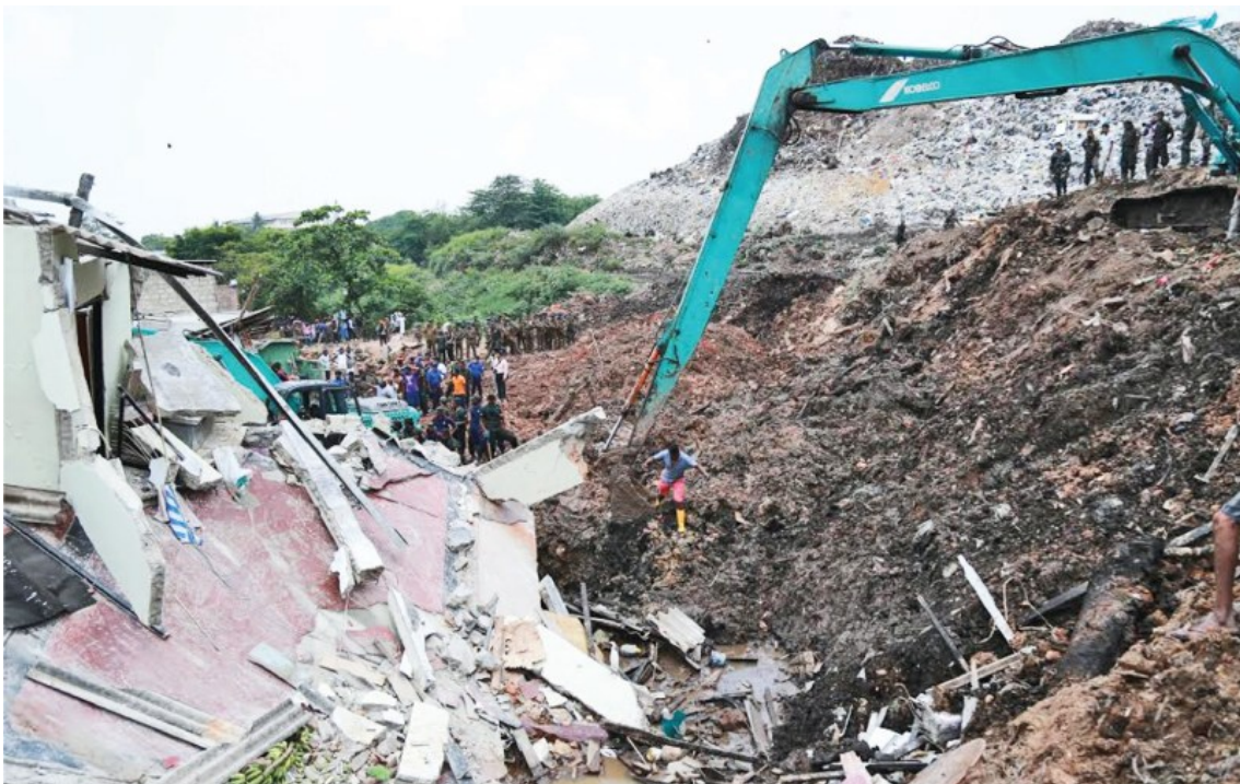
Figure 2-12: Aftermath of Meethotamulla MSW landfill failure (Disaster Services, 2020).
