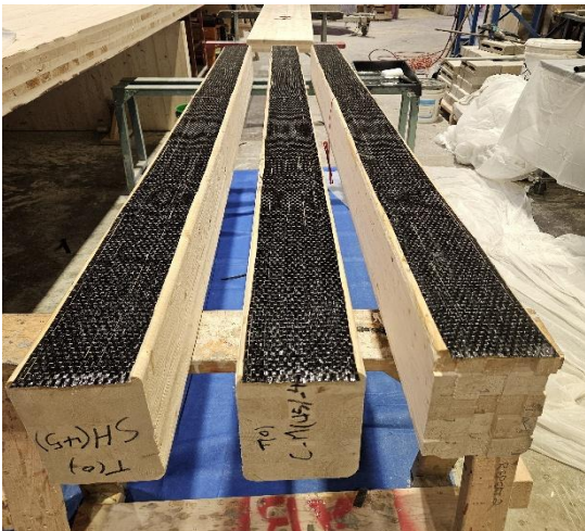
c) CFRP application along the tension side (Glulam beams)
