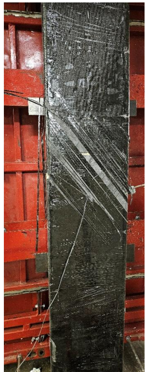
c) Tearing of fabric on tension side
