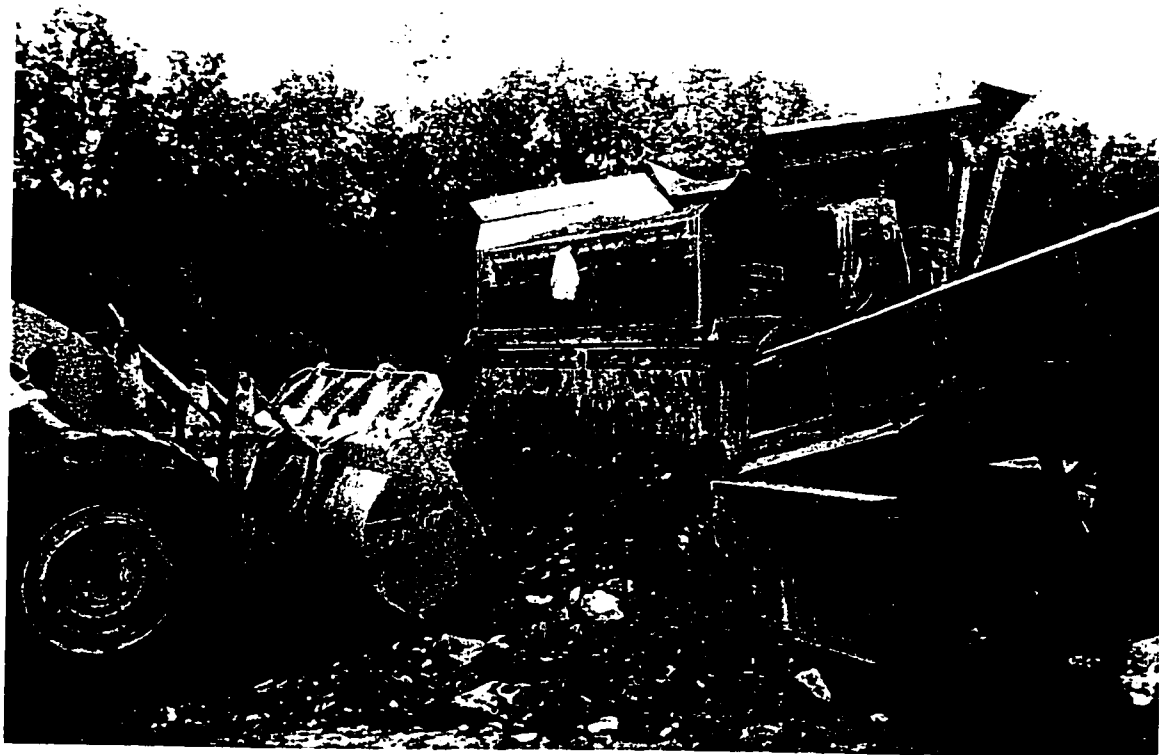
Figure E.3 - Screening Contaminated Soil.
