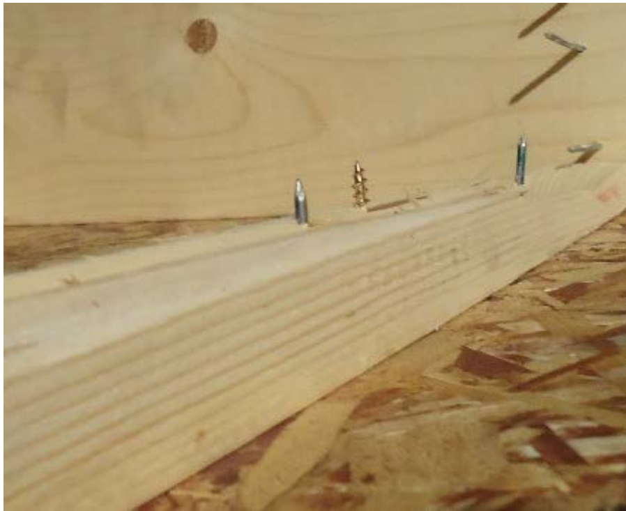
Figure 6.2 : Failure line with presence of nail and screw tips
