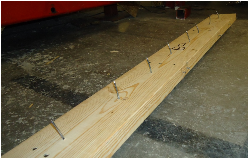
Figure 6.12 : Nail-withdrawal failure at bottom plate for Wall 18 Shot 1
