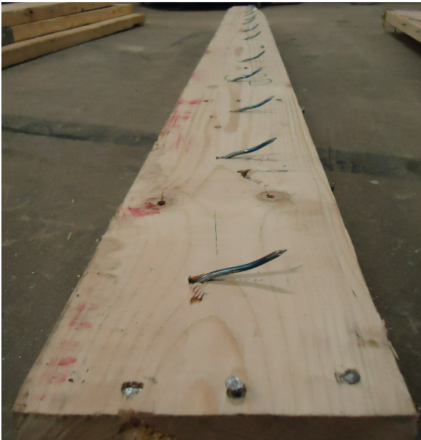
c) Nail yielding and withdrawal at bottom plate
