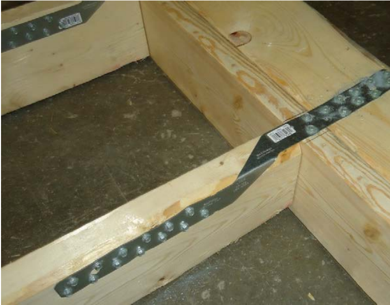
A. Installation of LTS18
