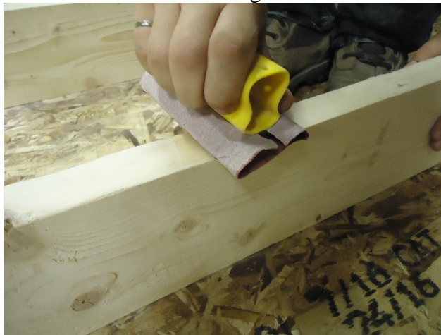
C. Sanding of dried epoxy
