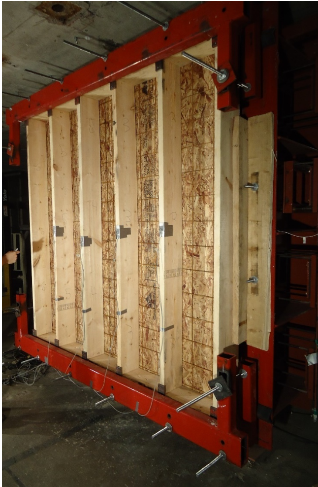
A. WWM as sheathing reinforcement
