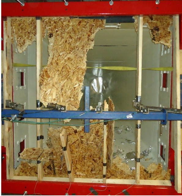
A. OSB wall with noticeable sheathing failure
