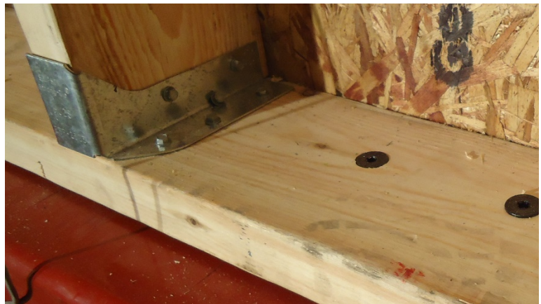
B. HU28 connection detail
