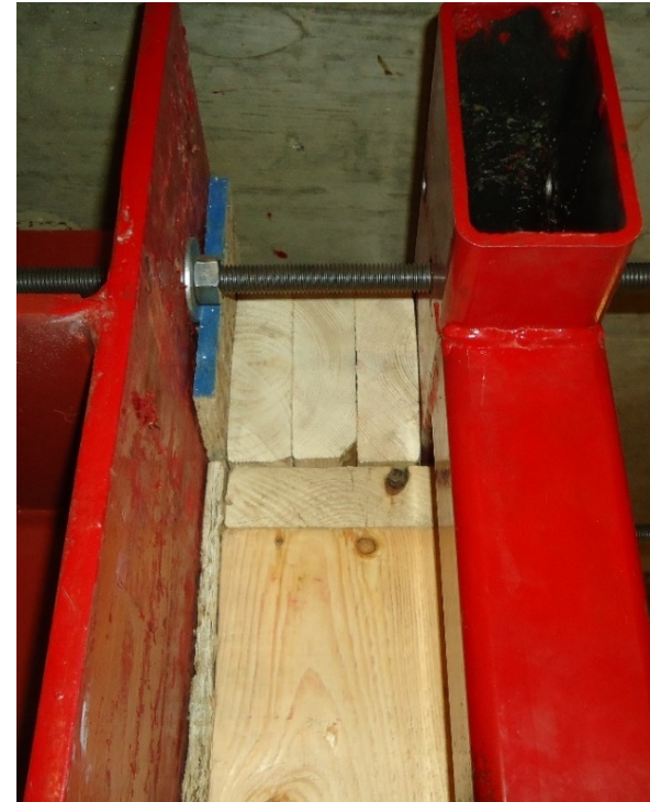
C. Close-up of top-plate-to-blocking detail (side-view)
