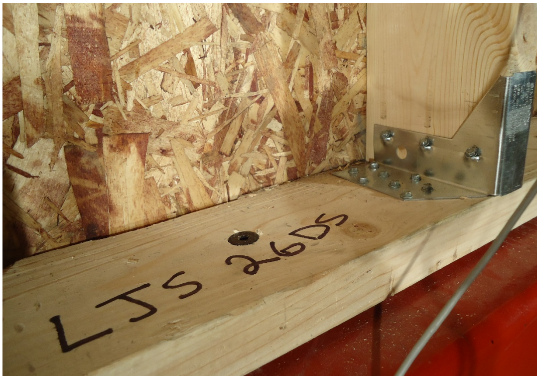
Figure 6.17 : LJS26DS connection detail
