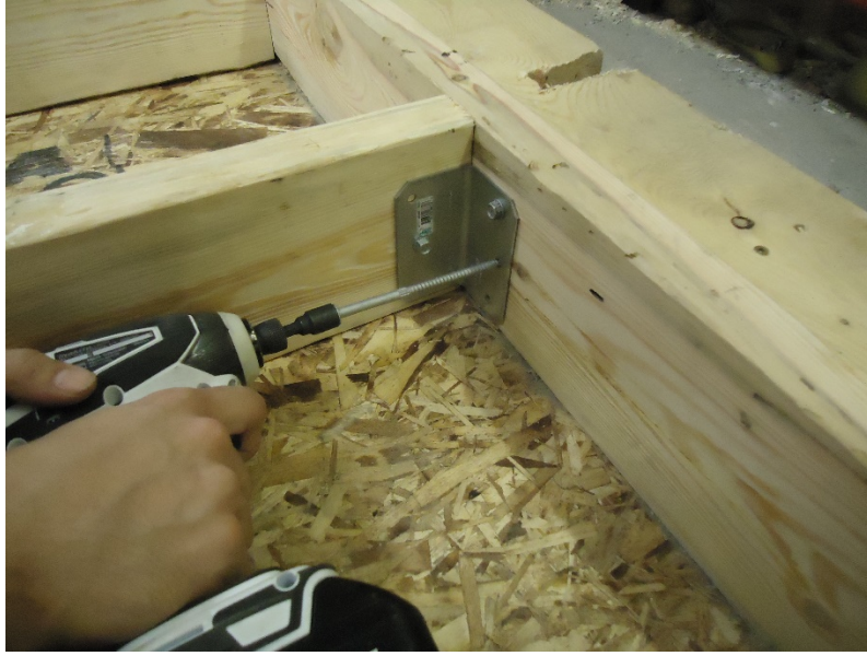
Figure 6.20 : Installation process of ML24Z connection
