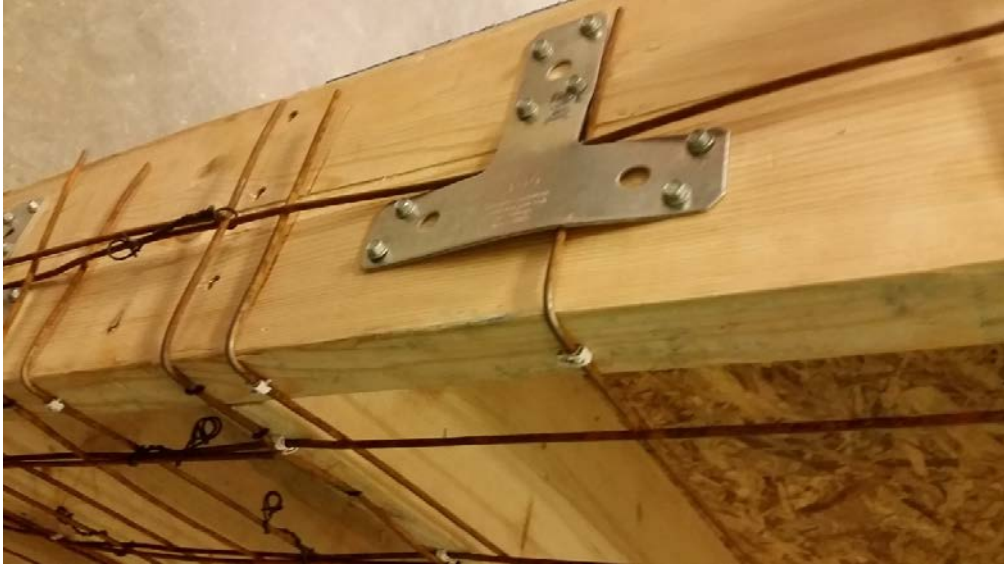
Figure 6.24 : Top-plate connection for WWM
