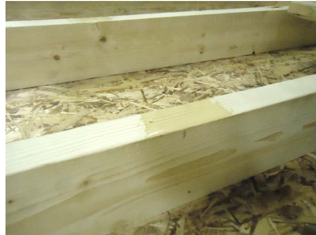
B. Application of epoxy
