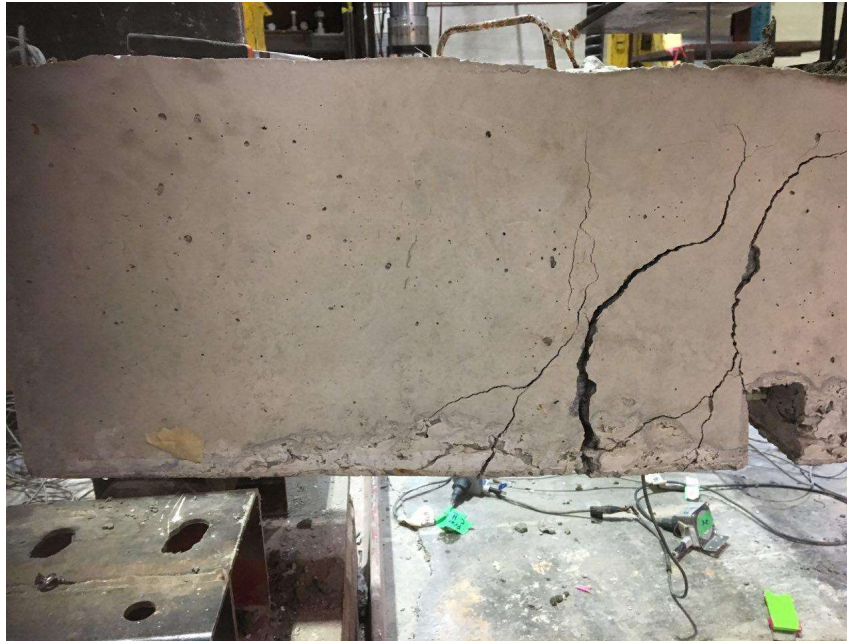
Figure 4.12 Shear Crack at Failure
