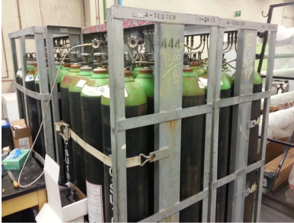
Figure 4.7: Driving Gas Supply
