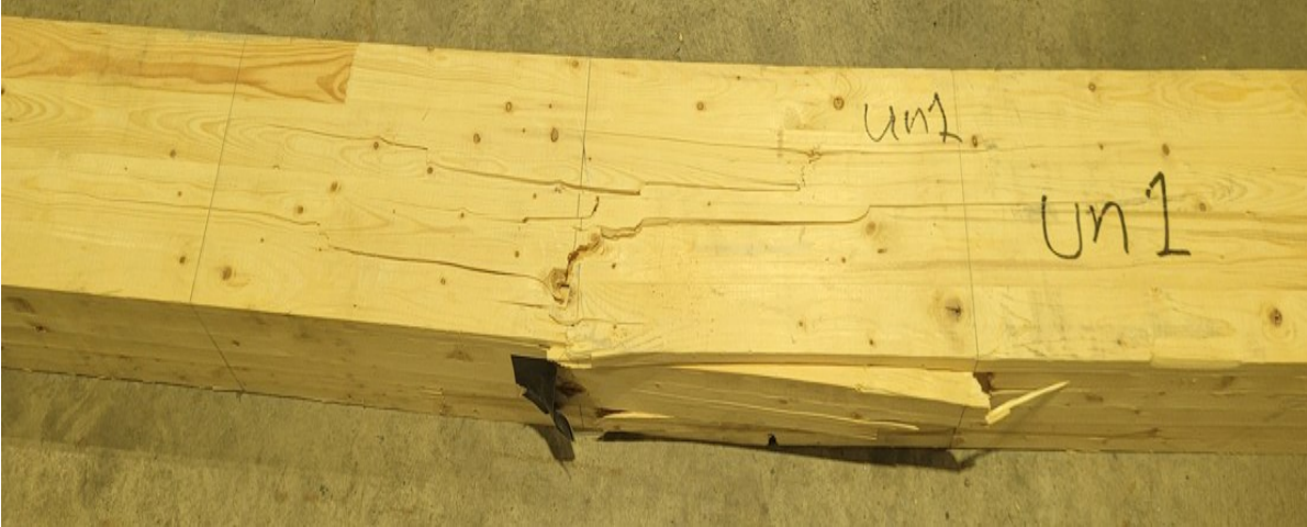
a) Damaged unreinforced beam
