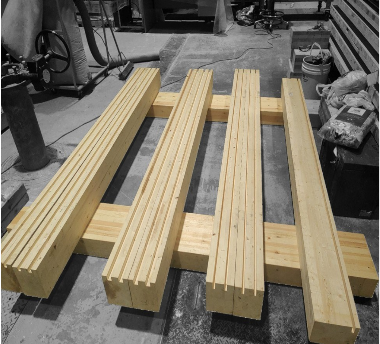
Figure 3.5: Glulam beams after drilling the grooves.
