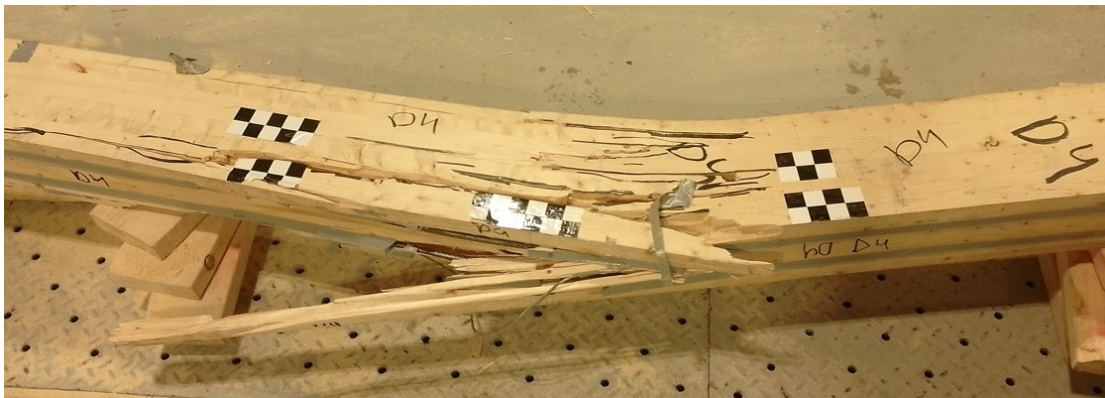
c) Damaged beam
