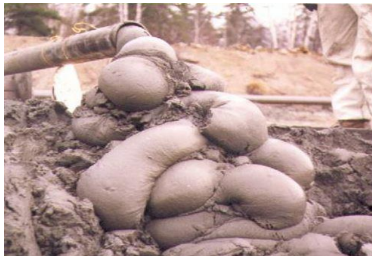
Figure 2.6: Cemented paste backfill being pumped (Hosseinzadeh et al., 2005)
