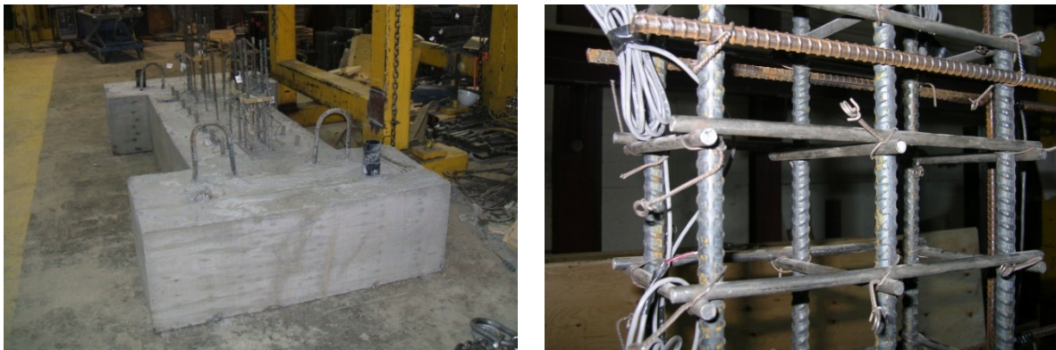
Figure 5.7 Shear Wall No. 1 during Construction
