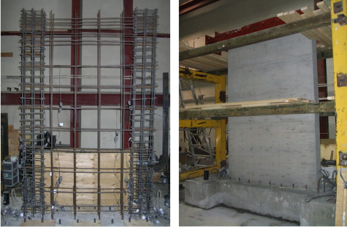
Figure 5.7 (Cont'd) Shear Wall No. 1 during Construction
