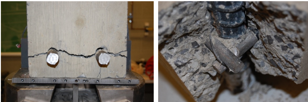
Figure 4.21 Typical Cracking and spalling of Concrete During Direct Shear Loading
