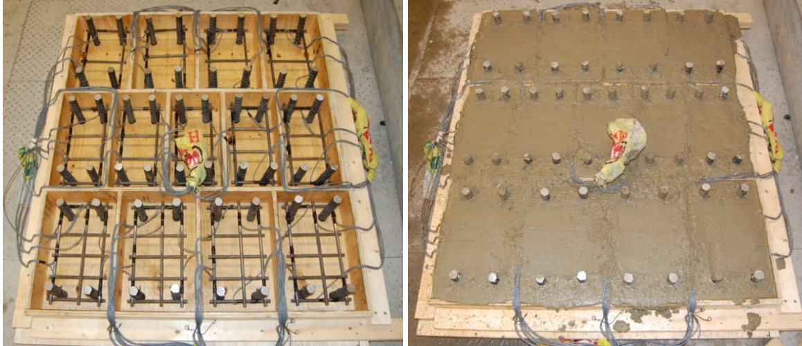
Figure 4.19 Cast-in Grid Steel Cage (Left); Freshly Poured Concrete Prisms (Right)
