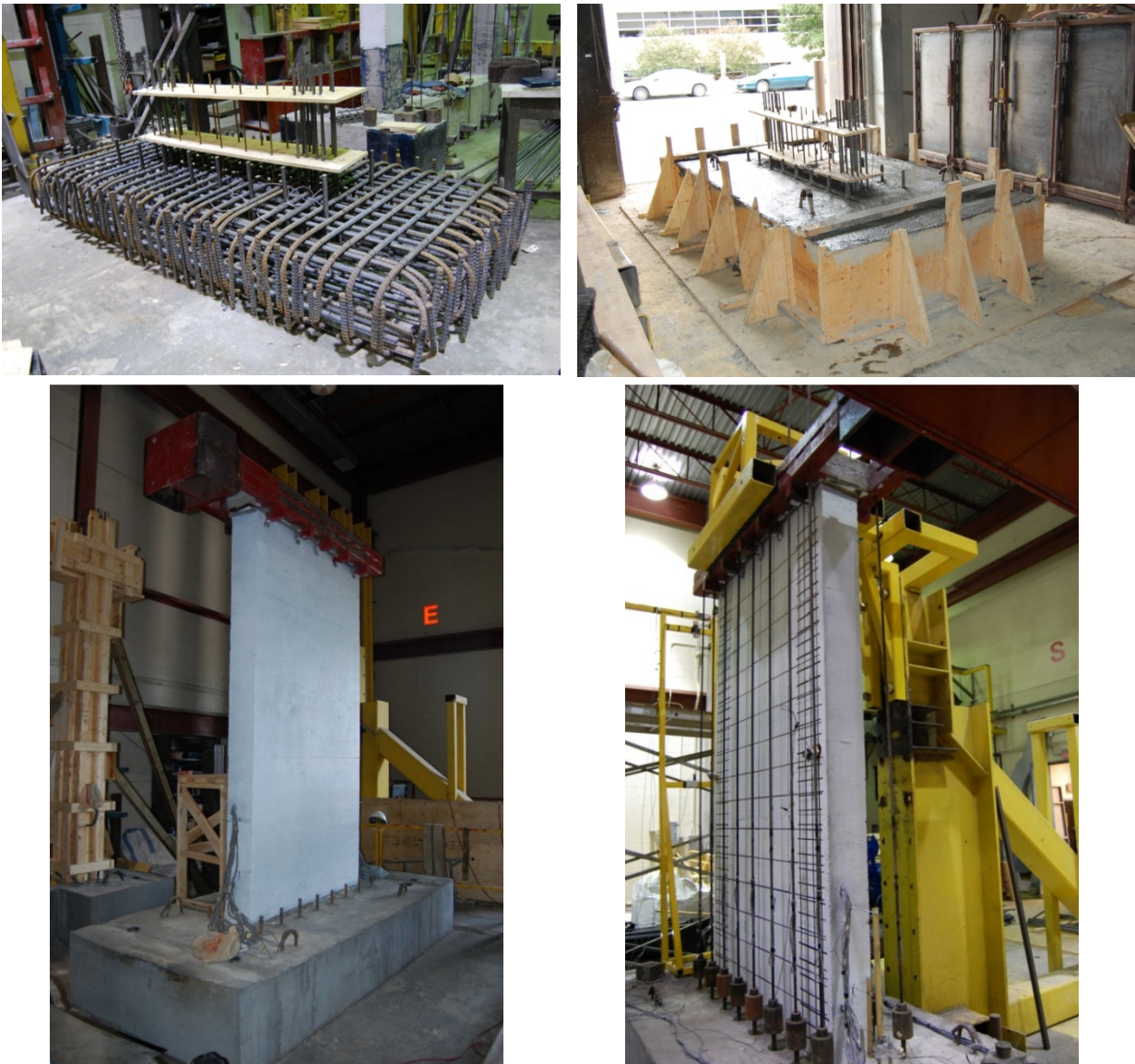
Figure 5.19 Shear Wall No. 2 during Construction
