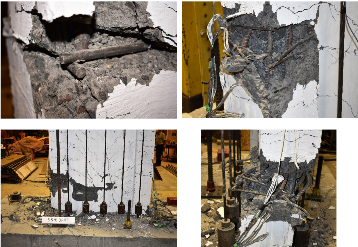
Figure 5.41 Shear Wall No. 3 Failure Photos
