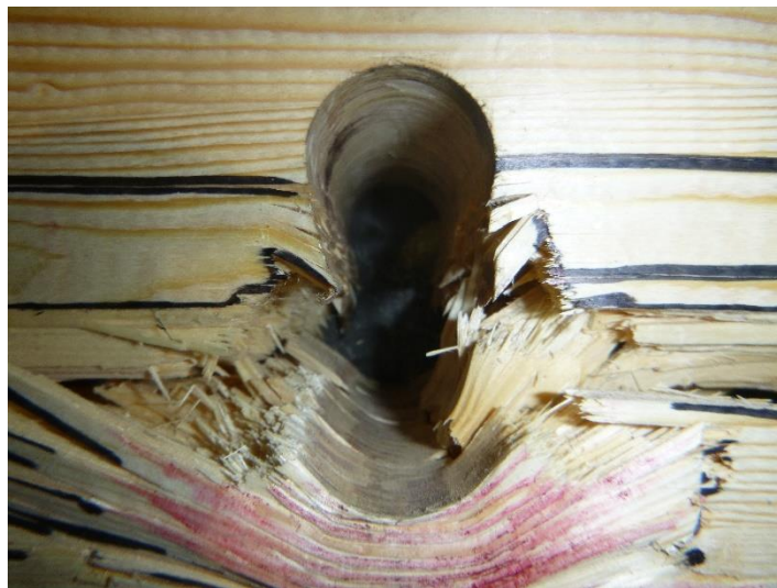
(b) Crushing in bolt hole
