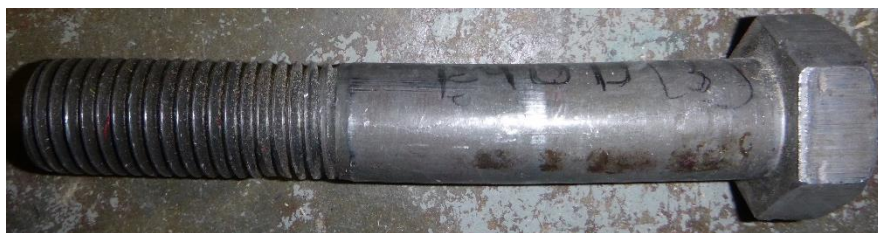
(c) Slight bending in bolt
