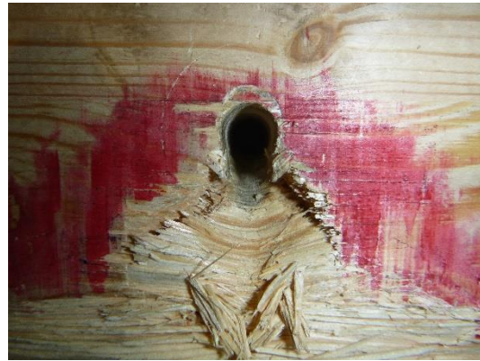
(b) Crushing at bolt hole edge
