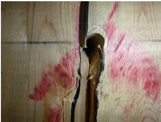
(c) Crushing at bolt hole edge
