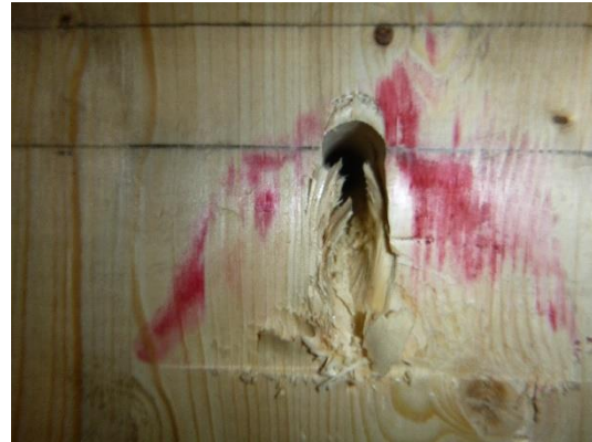
(b) Crushing at bolt hole edge
