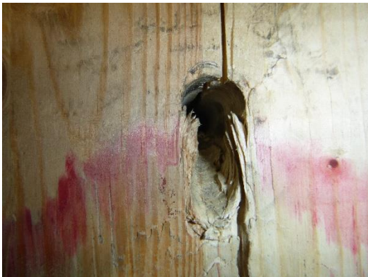
(c) Crushing at bolt hole edge
