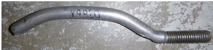
(c) Reinforced - sheared off bolt
