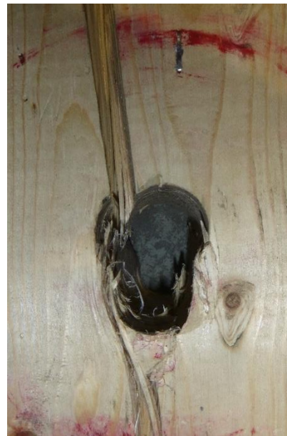
(b) Crushing in bolt hole
