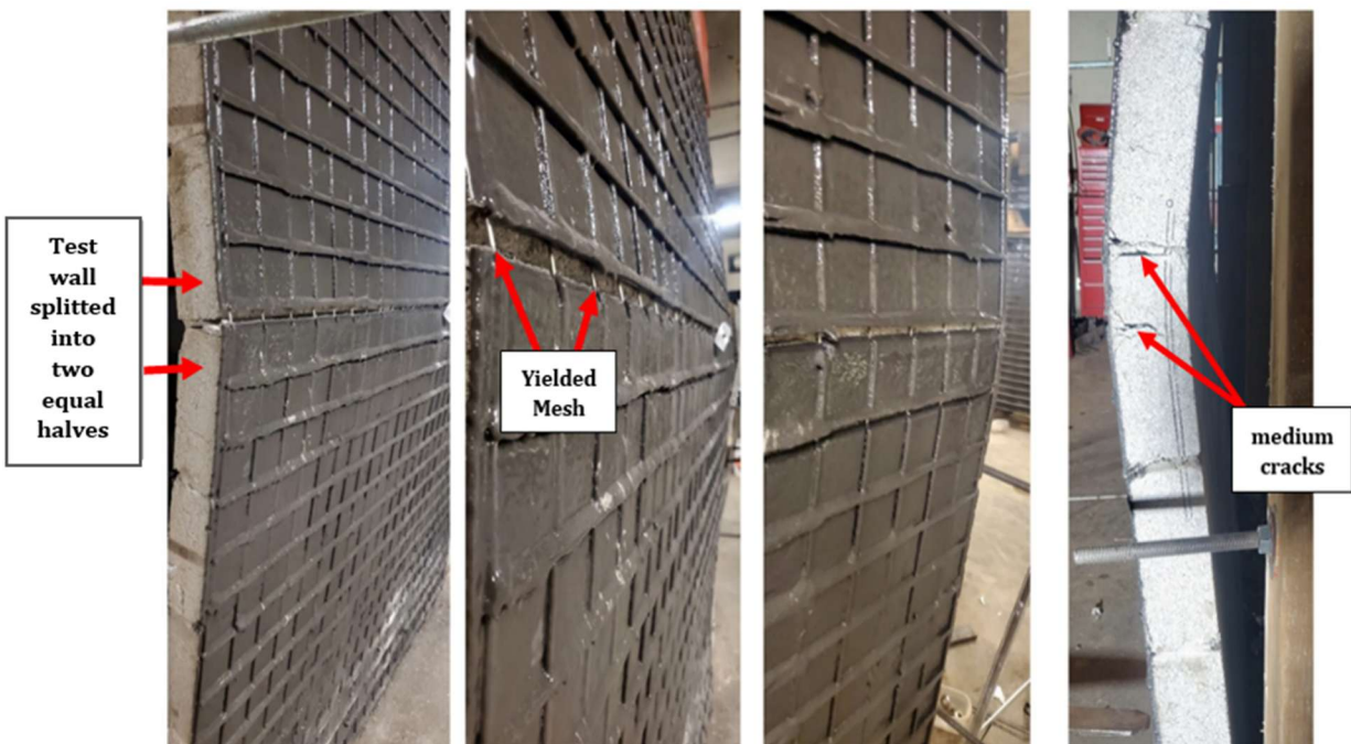
Figure 4.59. Failure of Wall-5-3
