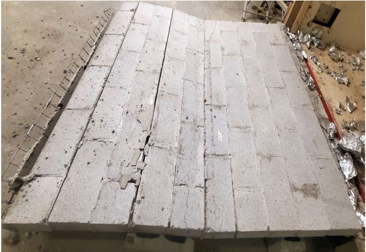
Figure 4.60. The exterior surface of Wall-5 after failure
