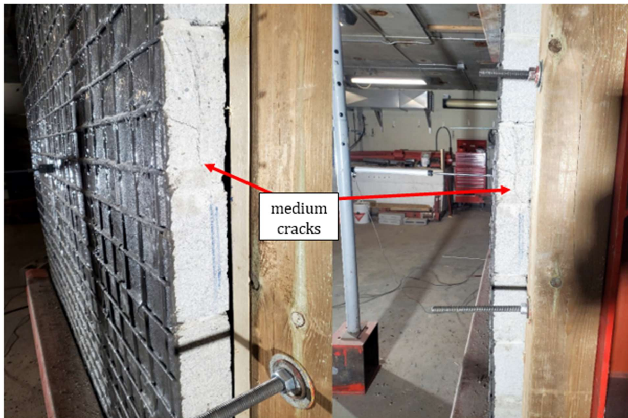
Figure 4.28. Medium cracks on the fifth course of wall-3-2
