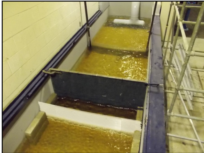
Figure 4-3: Turbulence Dissipating Baffles
