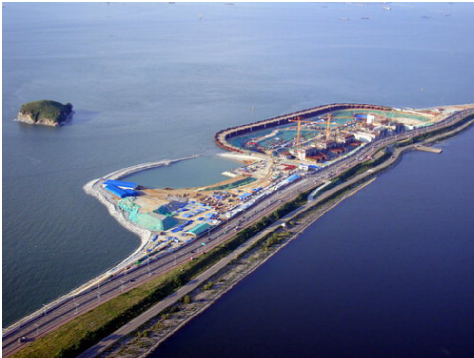
Figure 2-3: Sihwa Lake Tidal Power Plant under Construction, South Korea (Source: Wikipedia.org)
