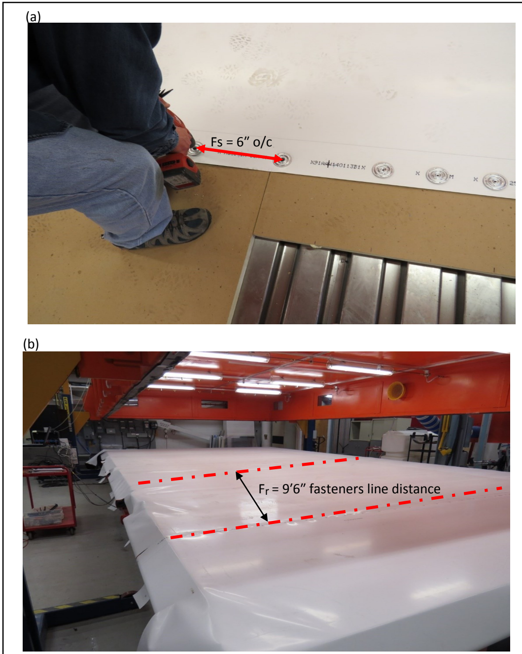
Figure 3.4 (a) Attaching membrane layer to steel deck, (b) Roof assembly
