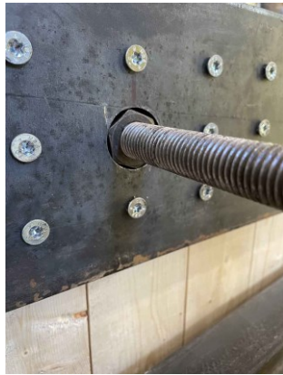
Figure 6-3: fitted connection between steel plates and treaded rods
