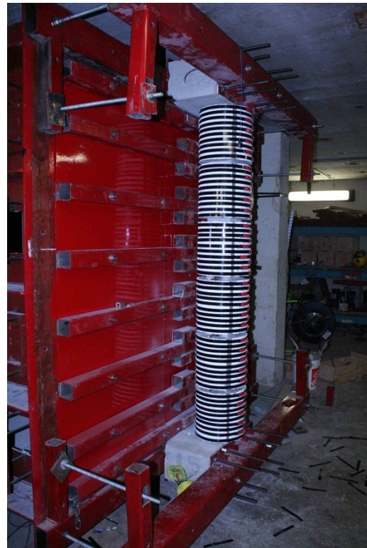
d) Completed Column
