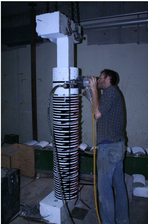
c) Installing Prestressed Strap
