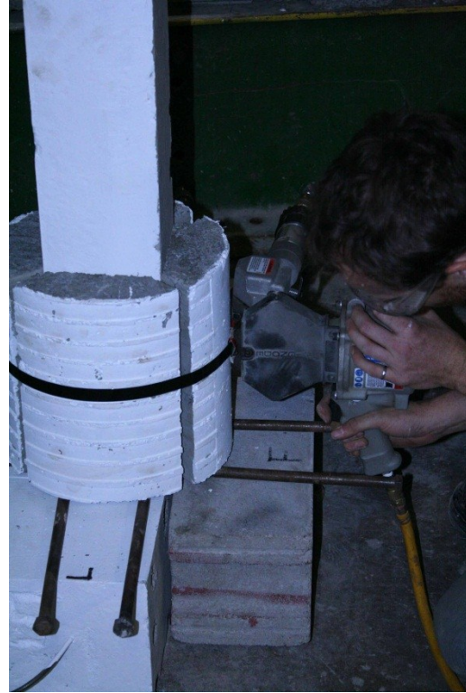
b) Installing Prestressed Strap
