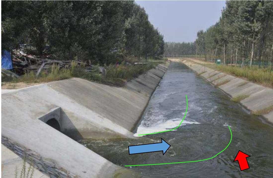
Figure 2. The confluence in Meixi Stream, China. The flow direction is shown as arrows: the blue arrow stands for the tributary flow while the red arrow stands for the main flow. The blue line indicates the shear layer. (Modified after [22])
