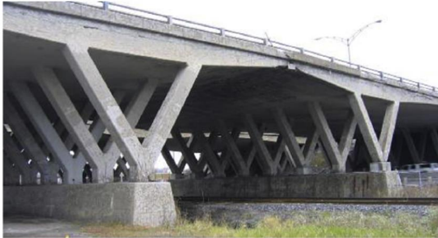
Figure 3.1: RBC overpass after nearly 50 years in service (Sanchez et al., 2020).
