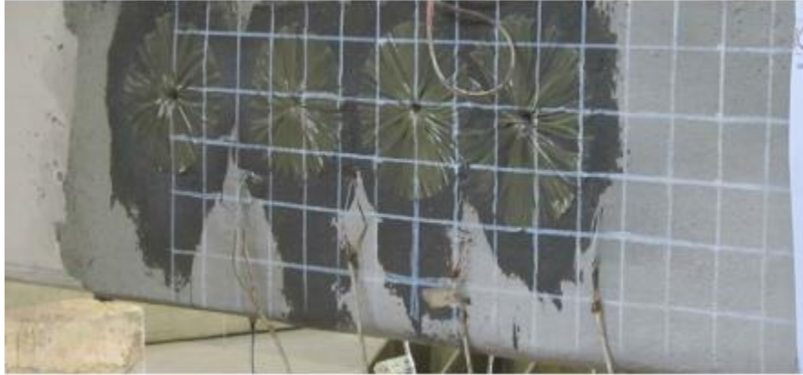
Figure 2.4: Spike anchors installed into the beams (Gonzalez-Libreros et al., 2017)
