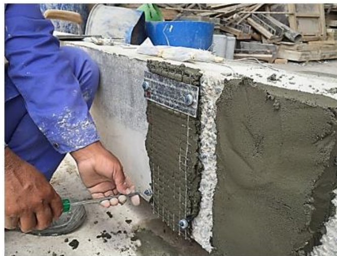
Figure 2.6: Mechanical FRCM anchorage (Younis et al., 2017)
