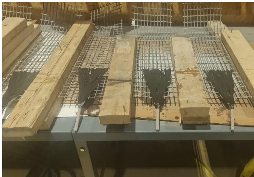
Figure 3.5: Carbon spike anchors installation
