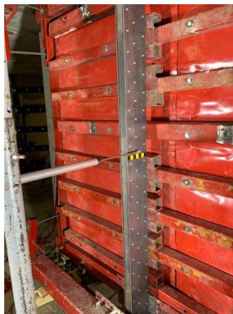
(e) Mullion 3H before test
