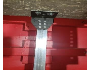
Brackets at top and bottom of slab at the top end of mullion
