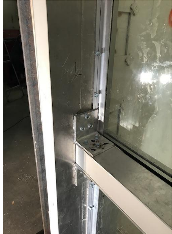
Figure 2.8: Mechanical glazing and mullion connection strengthening
