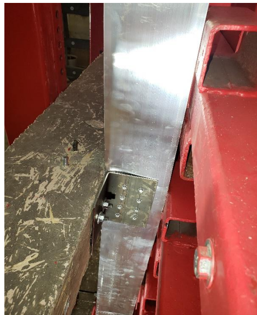
b) Loosened side bracket
