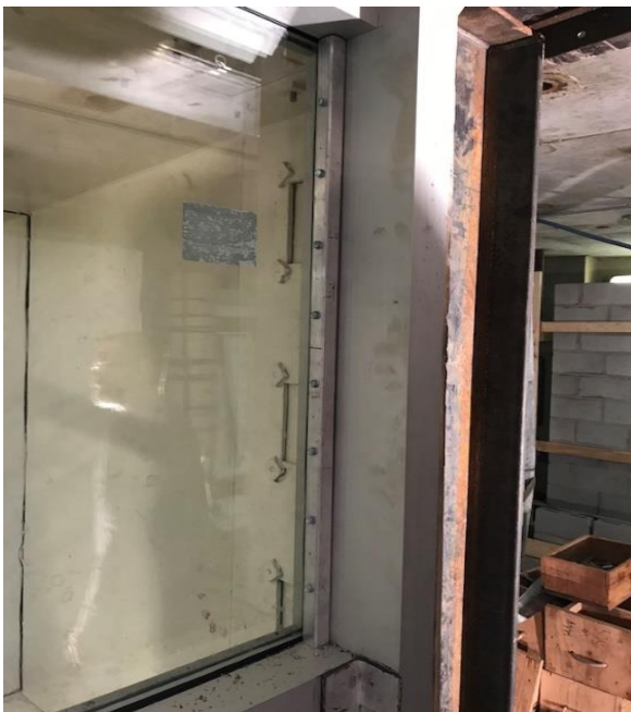
(a) Mechanical glazing
