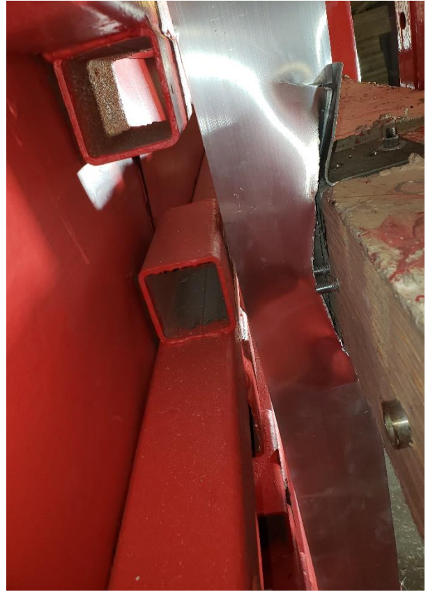
c) Close-up of failure
