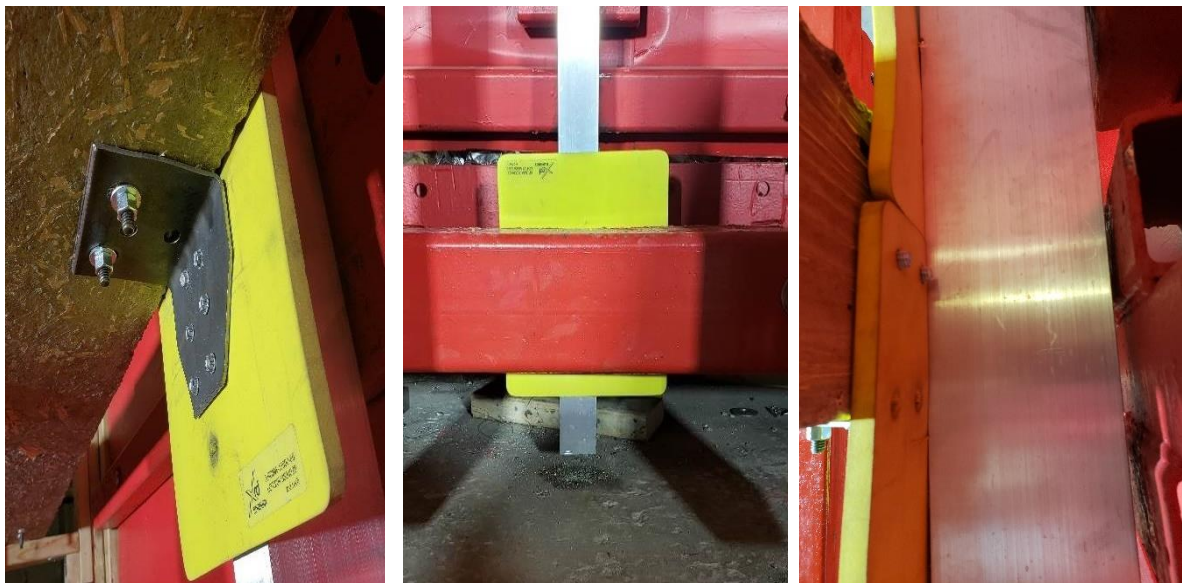
b) Inserted XRD rubber between mullion, concrete beam, and brackets
