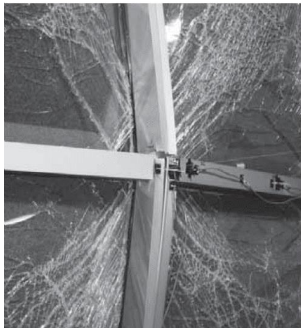
b) Loaded specimen just after mullion fracture
