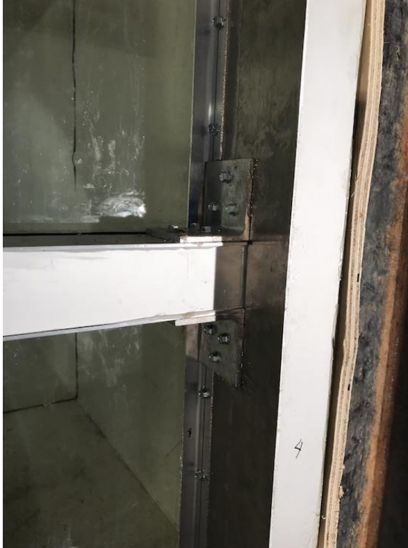
Figure 2.8: Mechanical glazing and mullion connection strengthening
