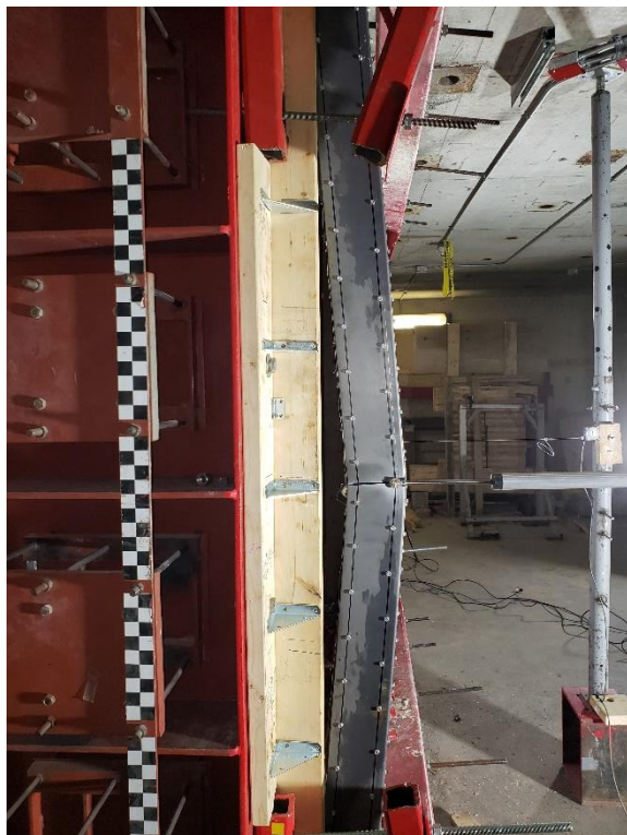
a) Mullion residual deflection
