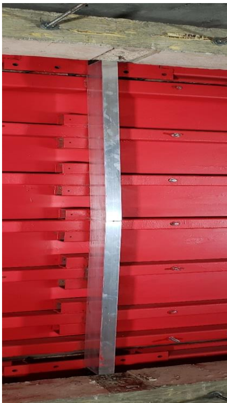
a) Overall view of single mullion
