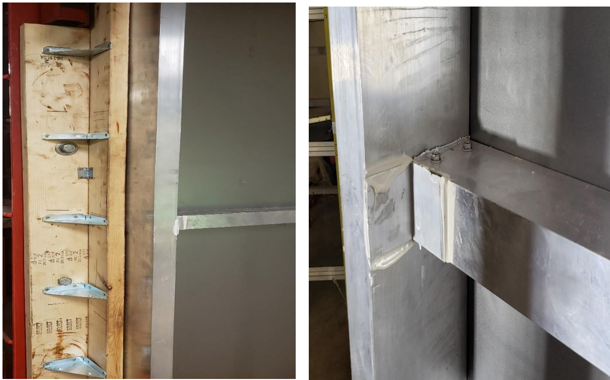
Figure 3.6: First curtain wall; without hardening of mullions, but with connections strengthened by epoxy glued aluminum brackets
