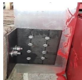
Brackets at the bottom slab edge connected to either side of the mullion web
