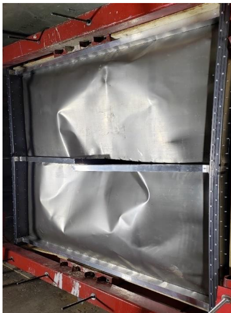
a) Overall curtain wall view
