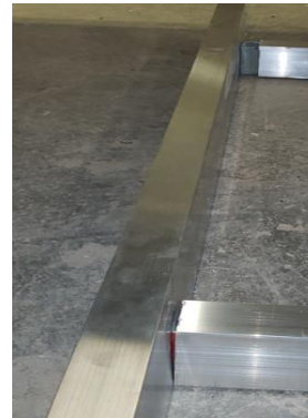
Figure 5.25: Mullion-to-transom connections considered.
