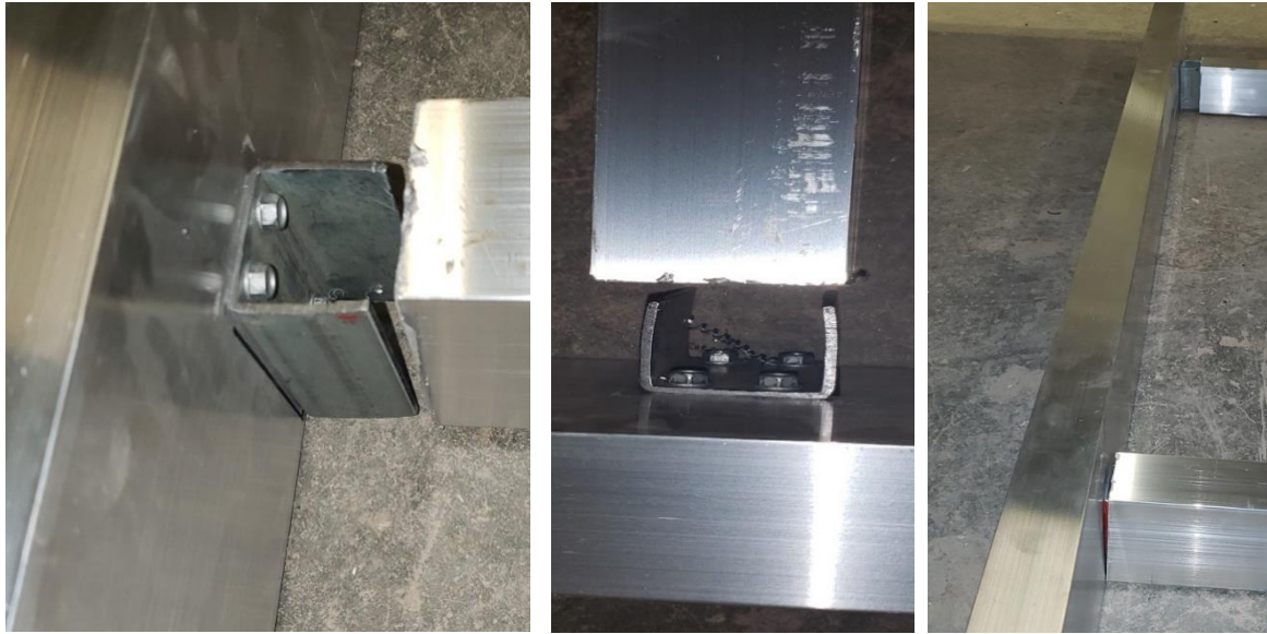
Figure 3.5: U-angle connections between mullions and transoms
