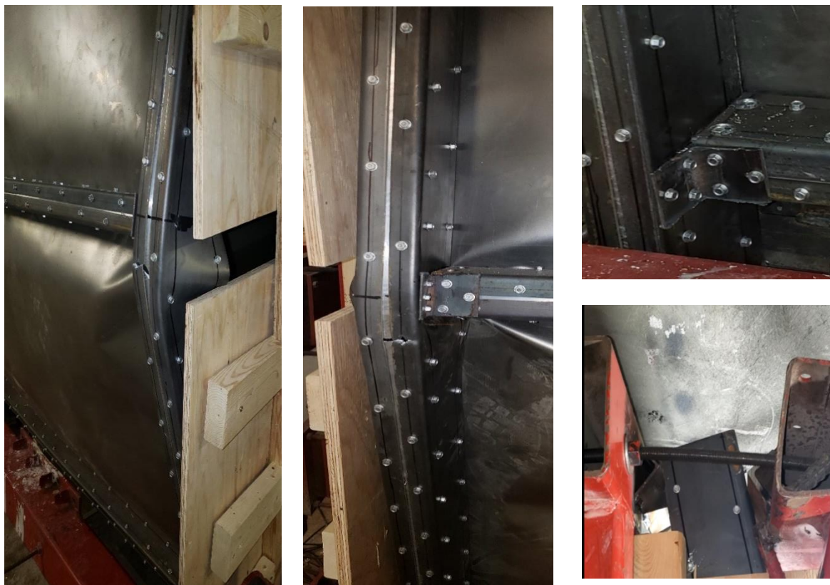
Figure 3.17: Third curtain wall, 2nd shot; after blast test.
