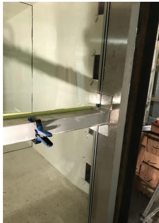
Figure 2.7: Application of aluminum plates and angles with epoxy adhesive for strength enhancement
