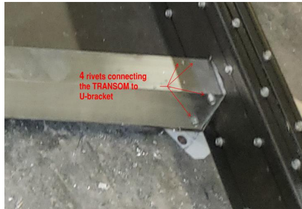
(b) Transom secured to U-bracket by 4 rivets
