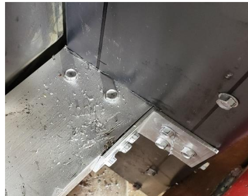
c) Anchored aluminum brackets
