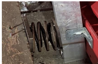
(e) Supports in (b)
