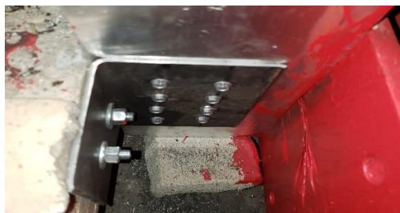
c) In tack side steel bracket
