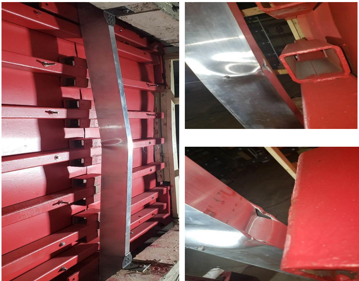
a) Overall view of mullion
