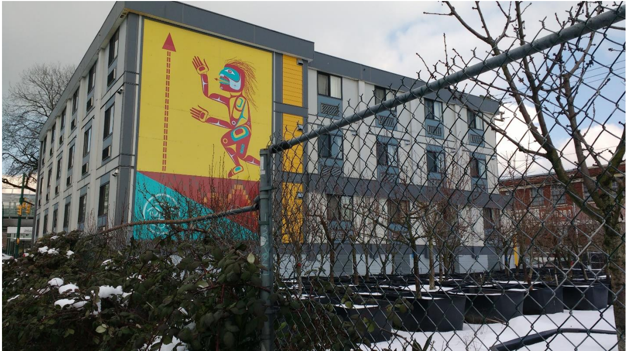
Figure 2. Temporary modular apartment units.
