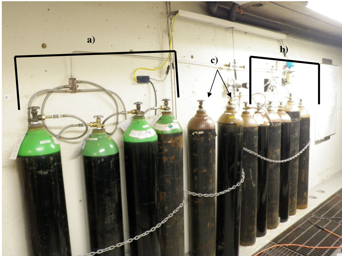
Figure 4.5: Photograph of the high pressure gas supply showing a) nitrogen driving gas bottles, b) helium driving gas bottles, c) helium feeding gas bottles
