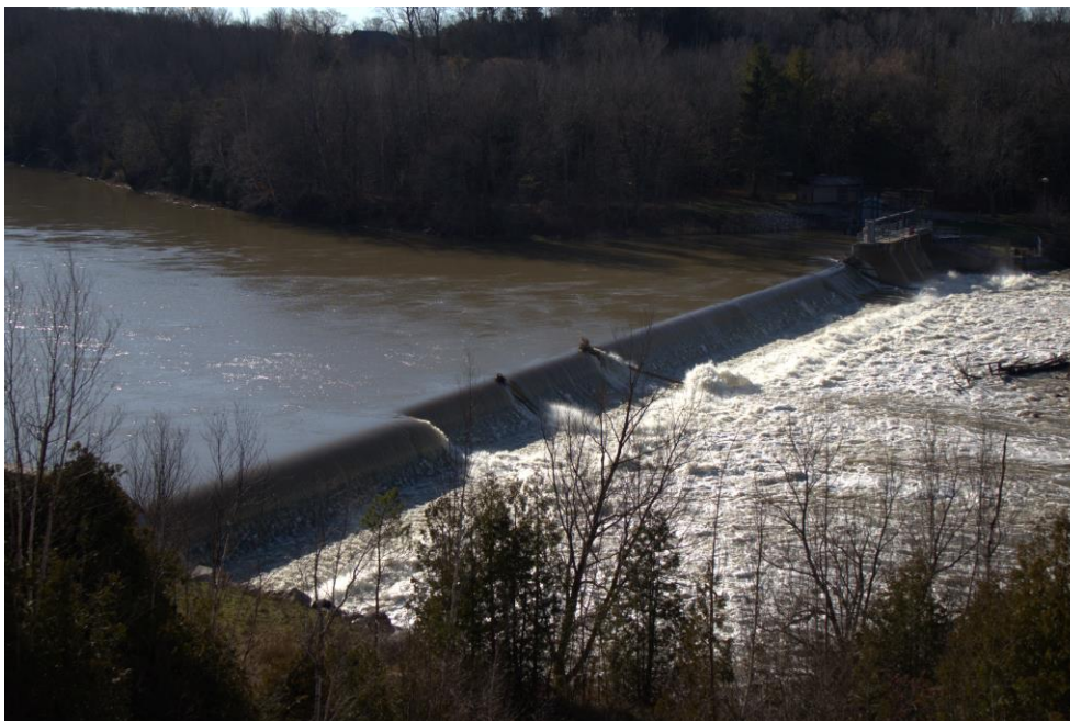
Figure 6. Top photo of Denny's Dam in Fall 2021
