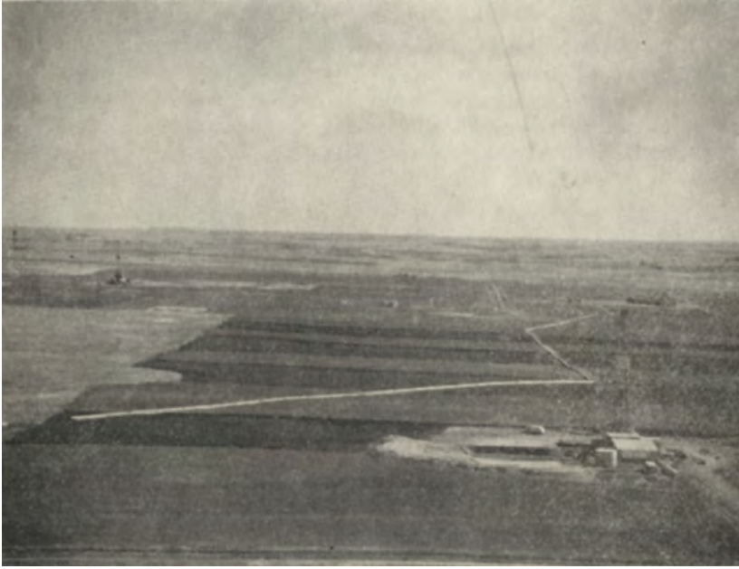
OIL WELLS AND PIPELINE NEAR TIOGA, N.D., SUMMER, 1954 — This is a representative scene of the major North Dakota oil producing area. The pipe line is the 24-inch line being laid to the Tioga refinery. Note that farming operations generally continue throughout the field. COURTESY GNDA
