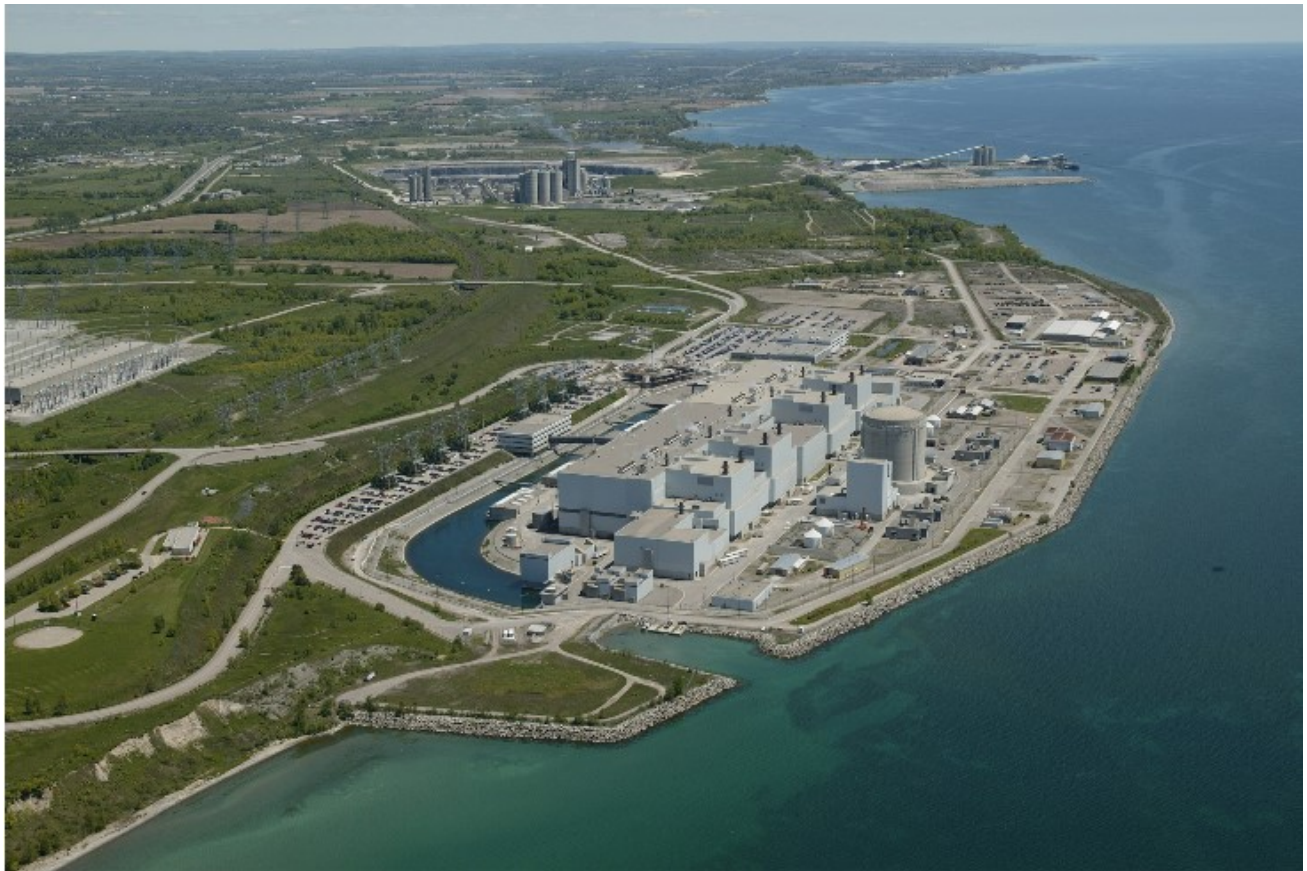
Figure 2.2. Ontario nuclear generating station ( http://assystem.files.wordpress.com )
