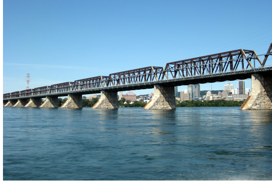
Figure 4.1: Study area: the Victoria Bridge in Montréal, Canada.
