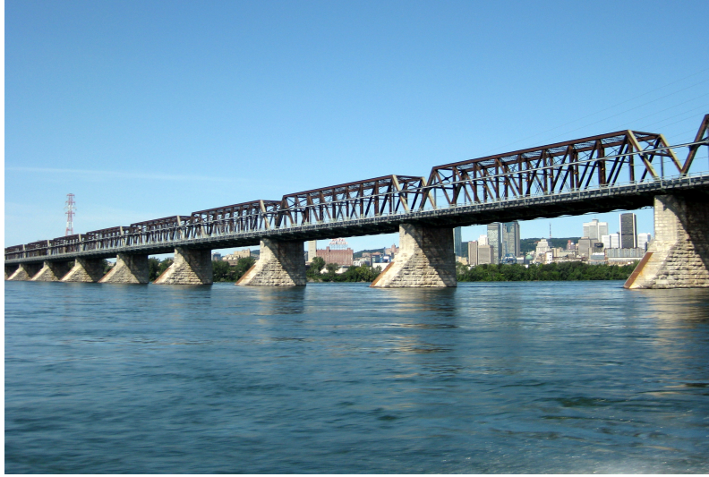
Figure 5.1: Study area: the Victoria Bridge in Montréal, Canada [88].
