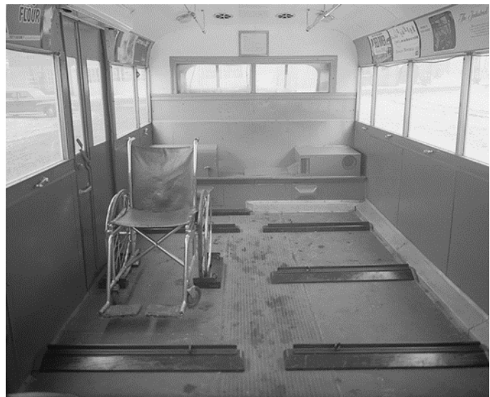
Figure 21: No. 574 Wheelchair bus converted from Model 23R Twin Coach, showing wheelchair securements, 6 January 1948. Credit: City of Toronto Archives, Fonds 16, Series 71, Item 15984
