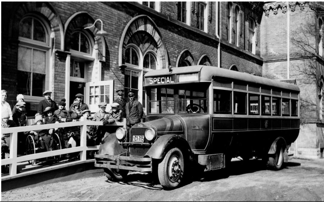
Figure 19: Adapted bus picking up children outside of Wellesley Street School, 15 April 1926. Credit: City of Toronto Archives, Fonds 16, Series 71, Item 4236
