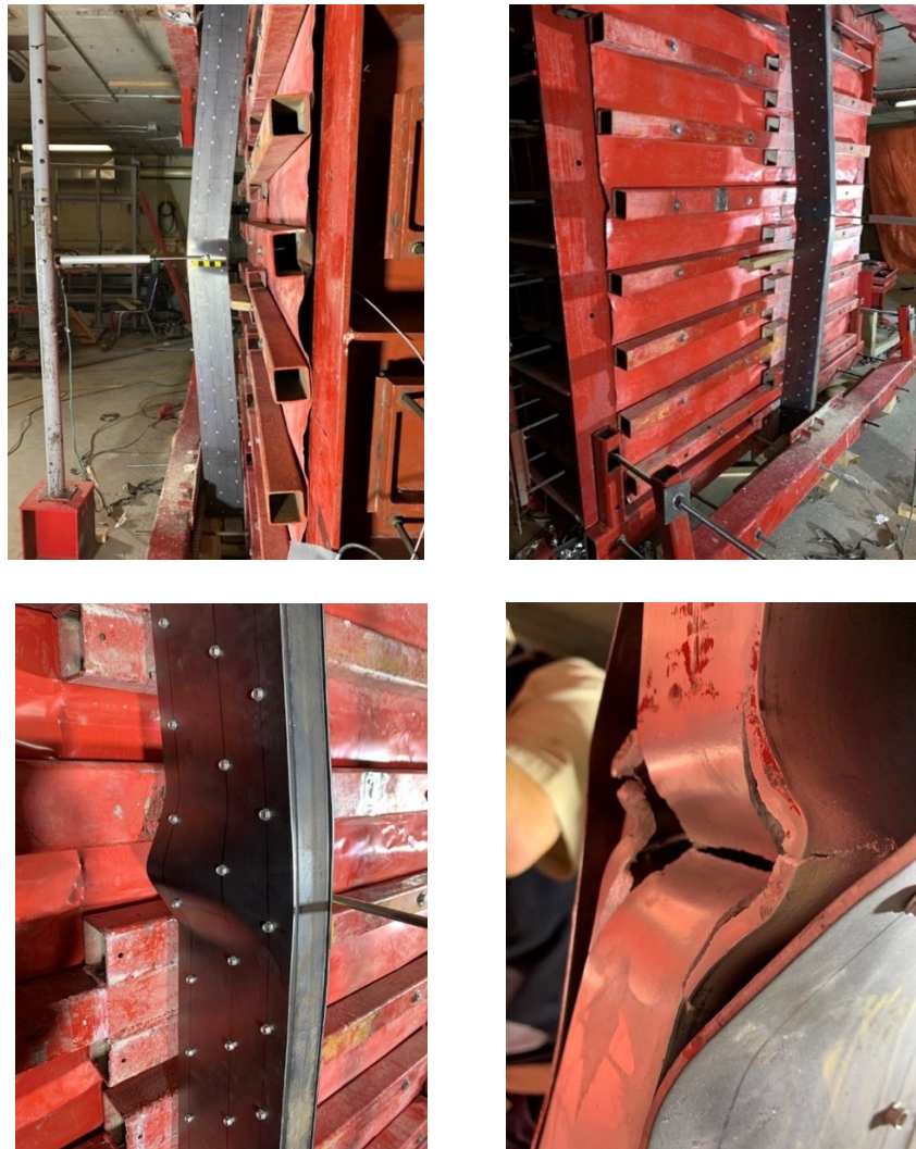
Figure 3 - 34 : Mullion 3H web buckling after second shot
