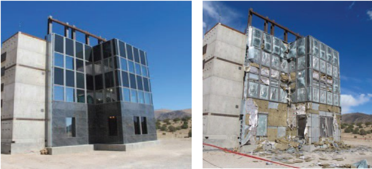
Figure 2 - 18 : SSCW before (left) & after blast detonation (right)
