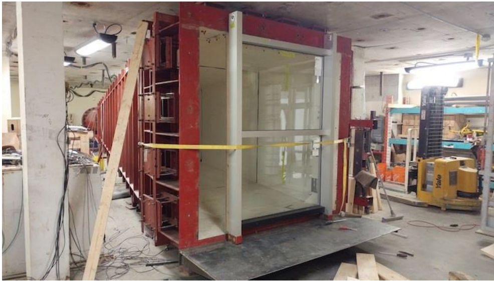
Figure 2 - 8 : Typical curtain wall specimen during installation for testing
