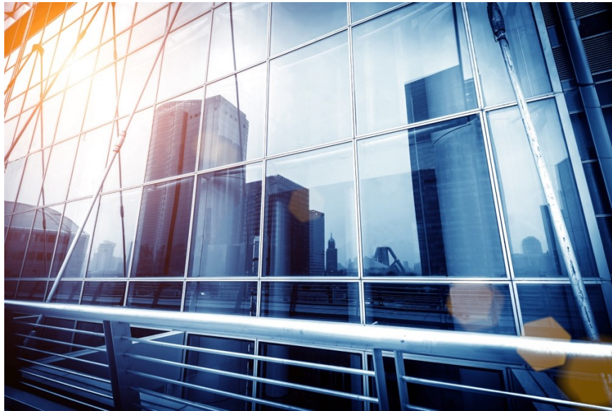
Figure 2 - 1 : Curtain walls with glass panels (Northview Inc. 2021)
