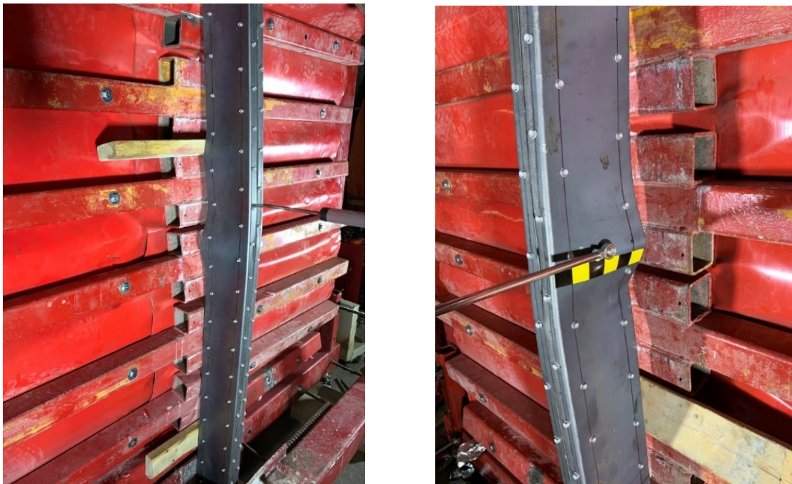
Figure 3 - 15 : Mullion 1H steel angle web buckling after the second shot
