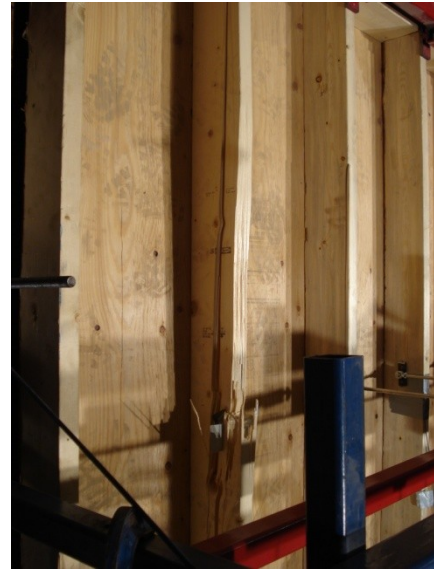
(b) Localized damage stud 2 and 3-Upper half
