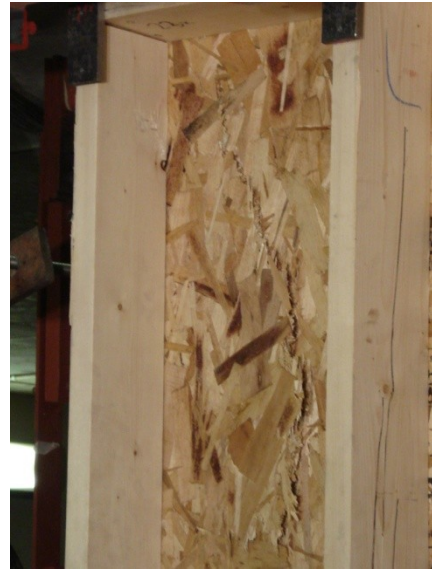
(b) View of sheathing failure
