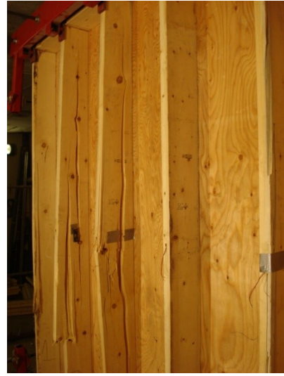
(b) Localized damage stud 1 to 3-Upper half
