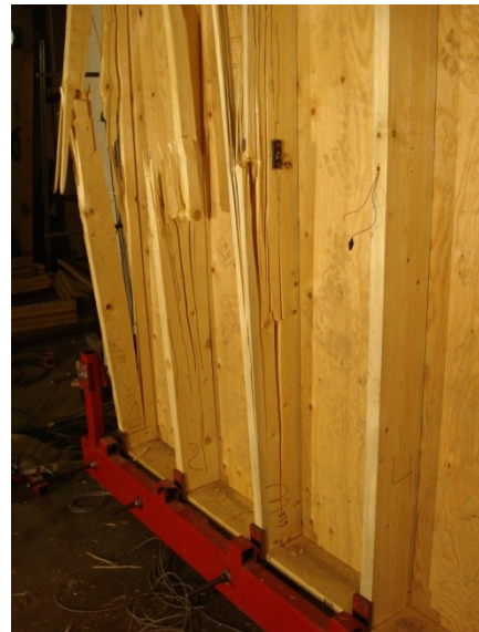
(c) Localized damage stud 1 to 3-Lower half
