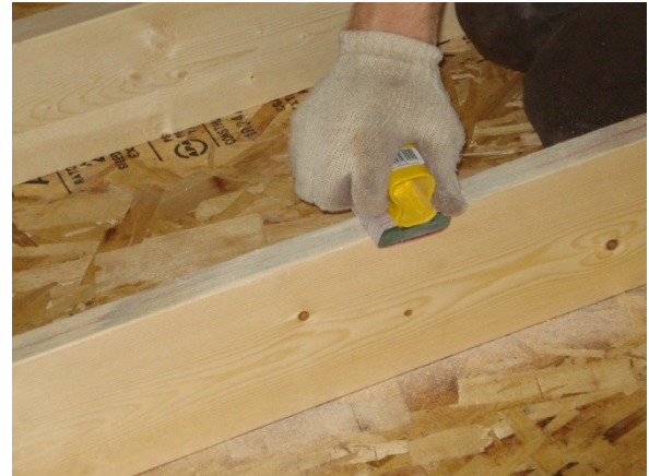
(b) Sanding epoxy layer
