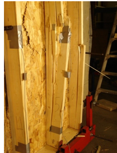
(c) Localized damage-Stud 4 to 6
