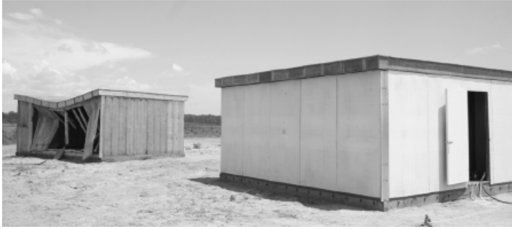
(a) Conventional and CSL building post blast
