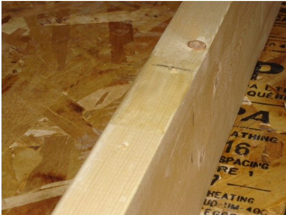
(a) Epoxy layer after sanding wood
