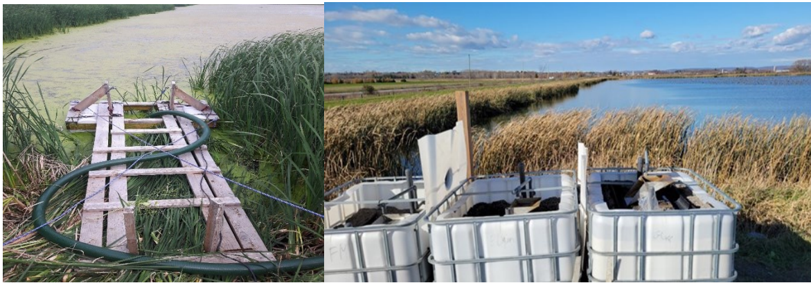
Figure 4.2 Pump Dock and Pilot Filters at Alfred Municipal Lagoon
