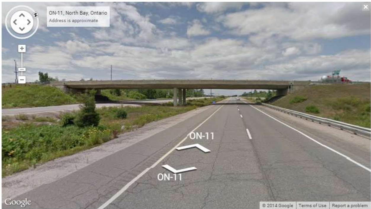
Figure 5. 1 Side View of the Actual Bridge (Google Earth™)
