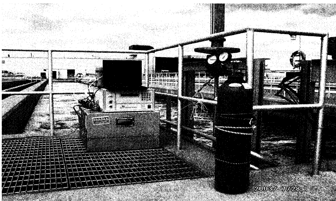
Figure 3.4 Total gaseous mercury sampling set-up over aeration basin (# 4) at ROPEC
