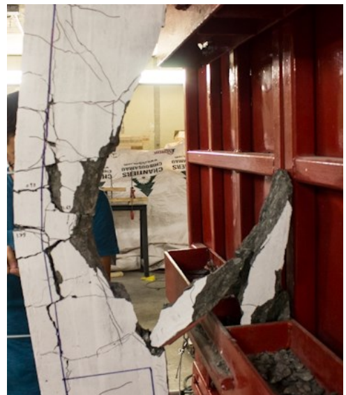
g) Mid-span crushing at Blast 4
