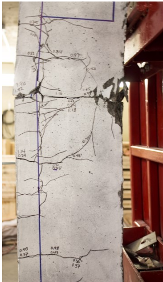
f) Mid-span cracking at Blast 4
