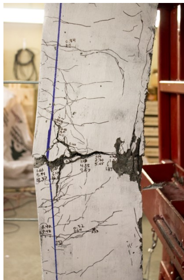
g) Mid-span splitting at Blast 5
