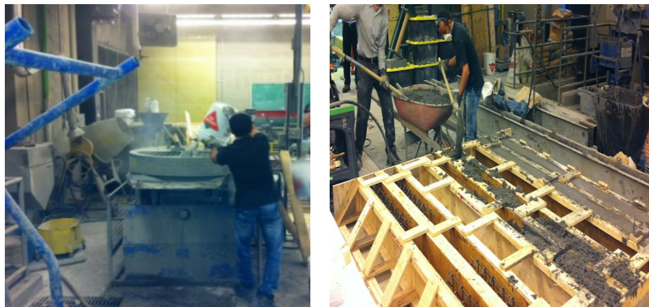
Figure 3-11 Concrete pan mixer and beams casting
