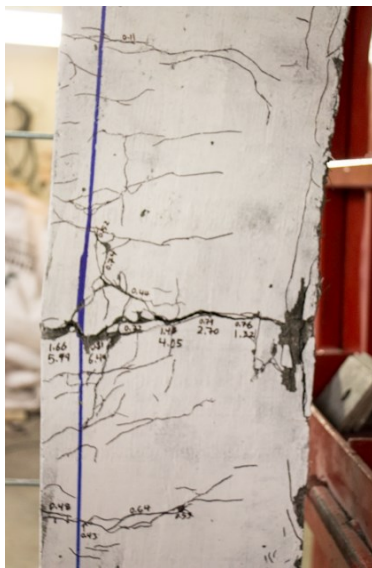
f) Mid-span cracks at Blast 4
