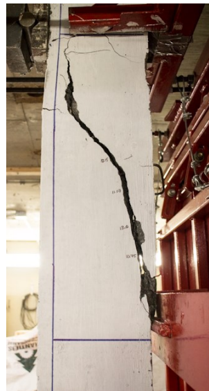
d) Shear-failure (top) at Blast 2, HSC-F0-20M-0
