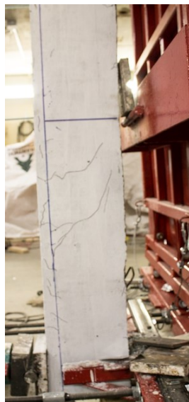
d) shear-span hairline cracks (bottom) at Blast 2
