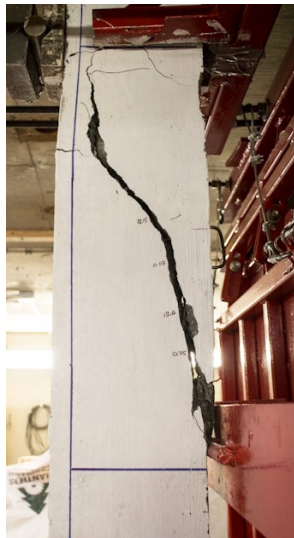
c) Shear-failure at Blast 2, HSC-F0-20M-0
