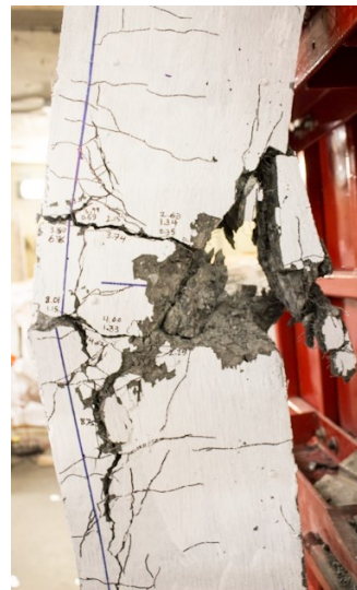
d) Mid-span crush & fibre pulled out at Blast 5, HSC-F1(ZP)-20M-S
