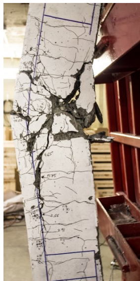
g) Mid-span crushing at Blast 5
