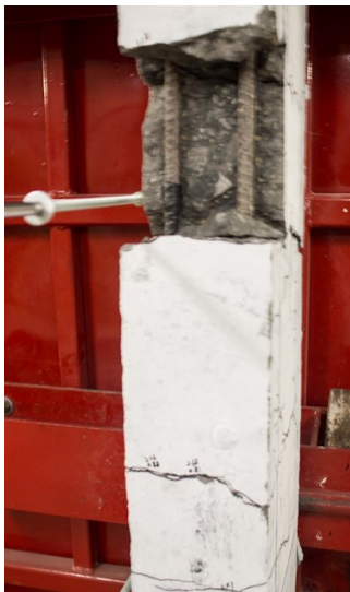
f) Mid-span spalling at Blast 2A, HSC-F0-#4-S
