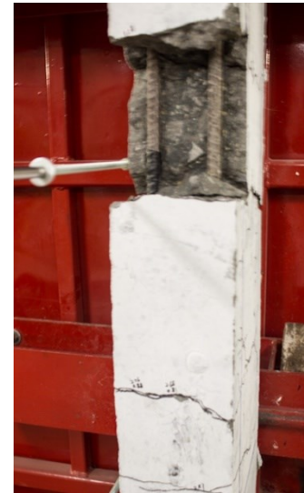
f) Mid-span spalling at Blast 2A
