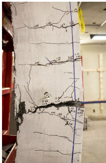
f) Mid-span splitting at Blast 4
