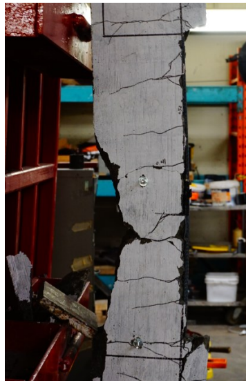
f) Mid-span crushing at Blast 3b
