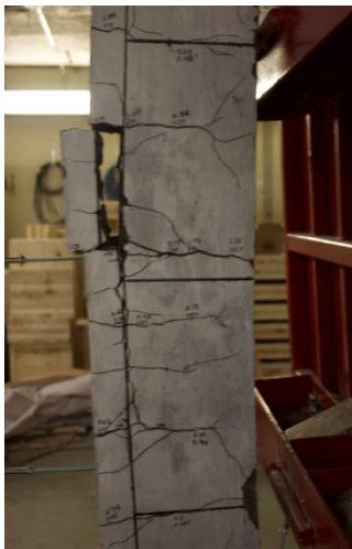
c) SCC-F0-#4-S-400 Mid-span spalling at Blast 3a (40 psi)
