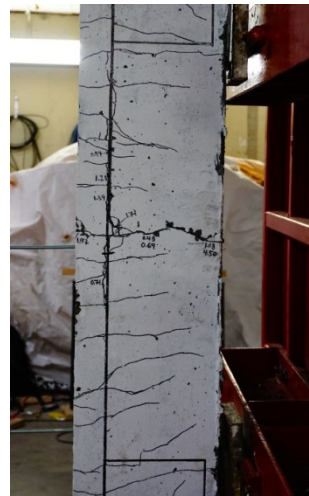
e) HSC-F1-#6-S Mid-span damage at Blast 4 (70 psi)
