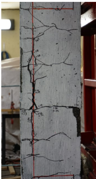
e) Mid-span cracking at Blast 3a
