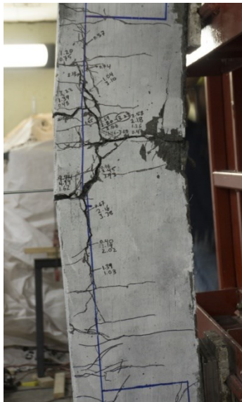
h) Mid-span cracking at Blast 5
