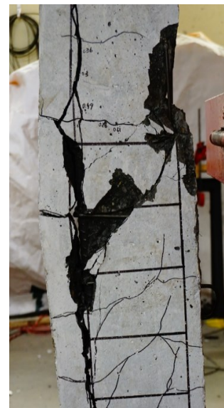
g) Mid-span crushing at Blast 4
