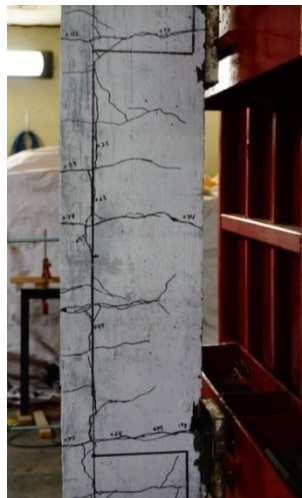
d) SCC-F0-#4-S Mid-span damage at Blast 3a (40 psi)
