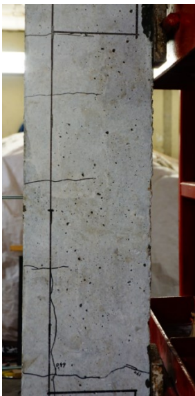
e) Mid-span cracking at Blast 2
