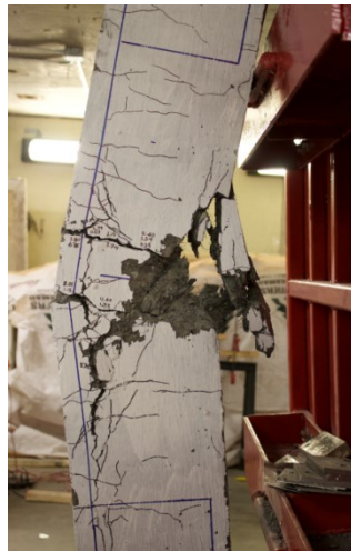
d) HSC-F1-20M-S-400 Mid-span failure at Blast 5x (80 psi)
