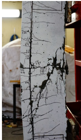
h) Mid-span cracking at Blast 5
