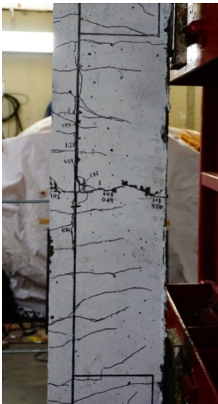
g) Mid-span cracking at Blast 4
