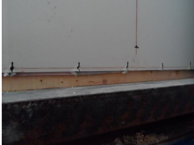
Figure 60: Wall 5-2 End Distance Failure
