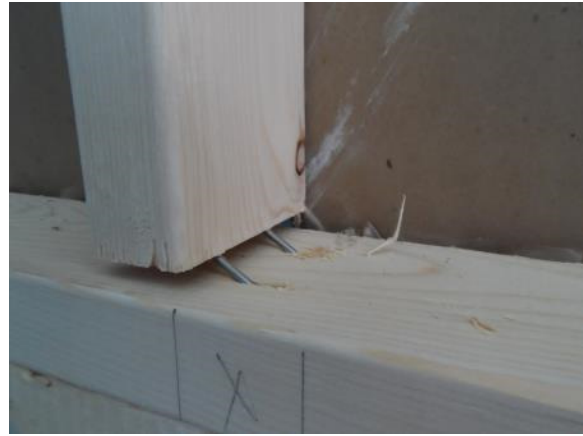
b) Wall 8-2 End Nails Yielding and Withdrawal
