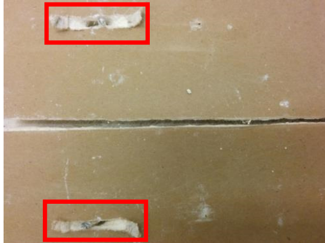
Figure 22: Gypsum Wallboard crushing
