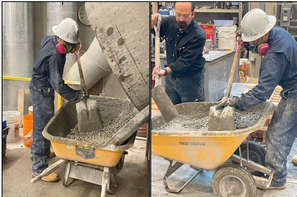
Figure 4-22: Concrete mixing of a 100-litre batch.
