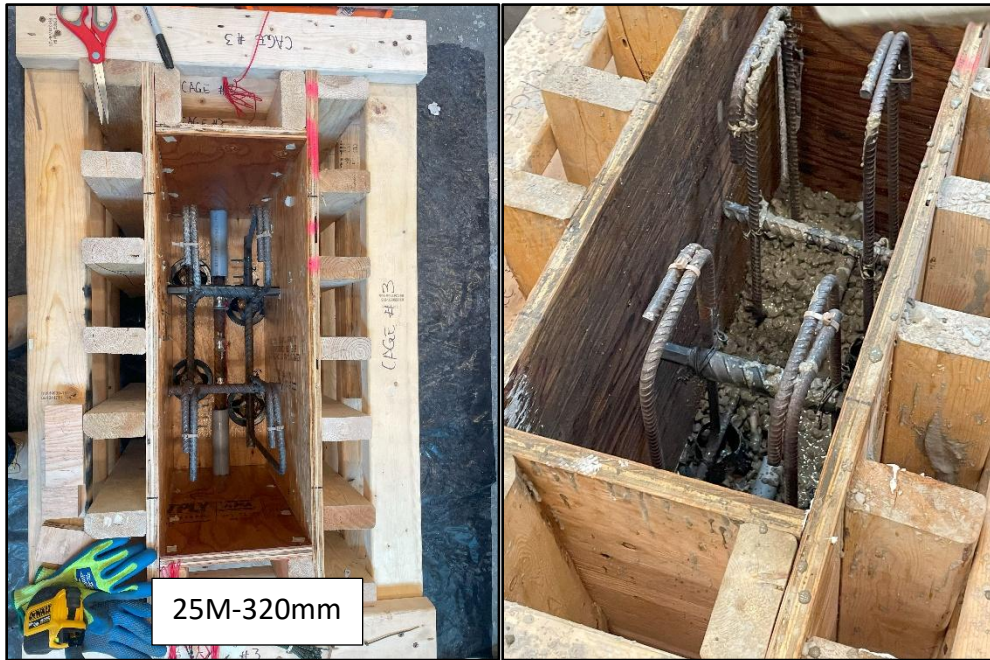
Figure 4-21: 25M reinforcing steel assembly of beam-end specimens.
