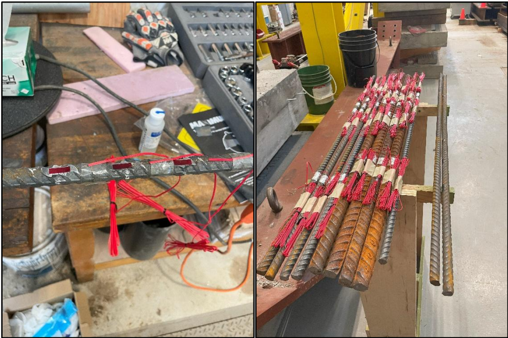
Figure 4-14: General use strain gauge installation (cables strapped for transportation).
