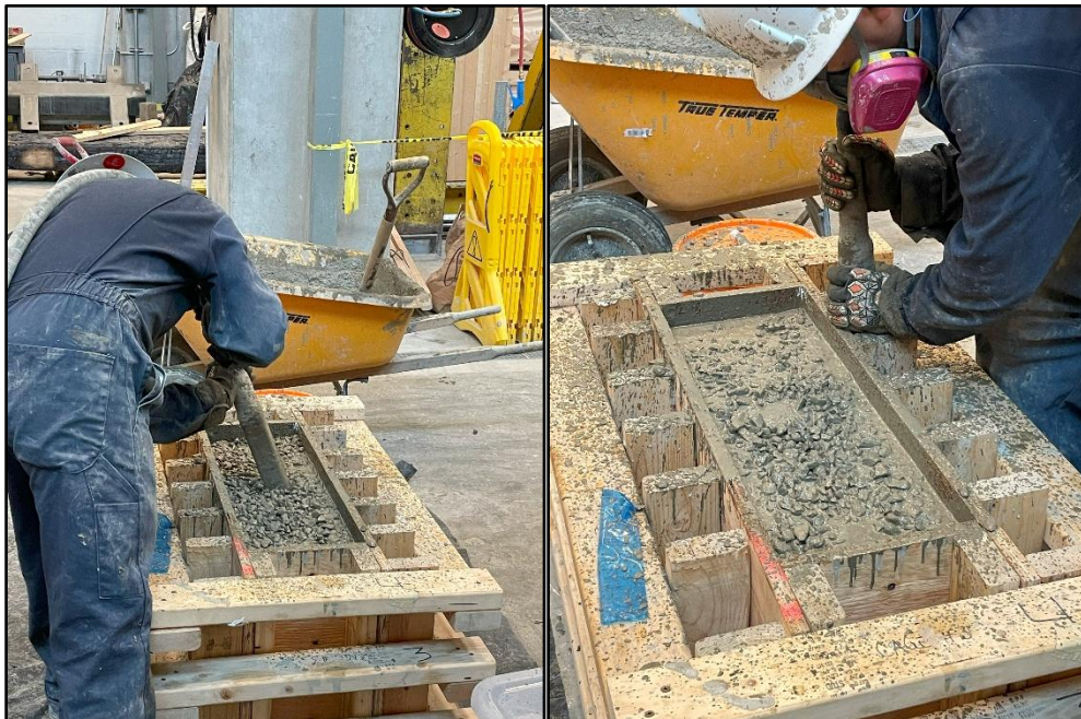
Figure 3-33: Vibration of structural specimens.
