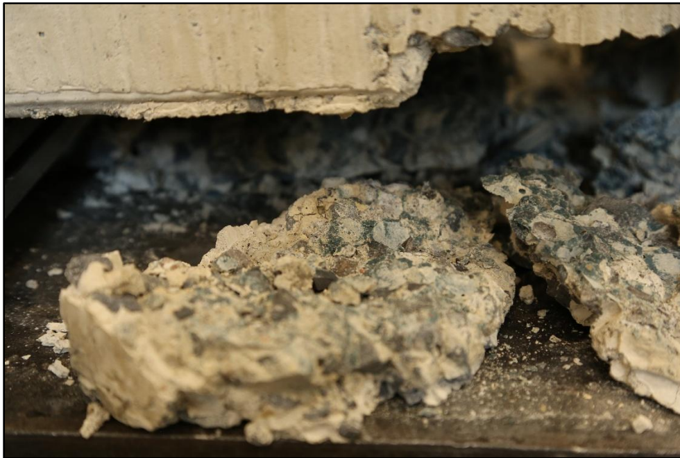
Figure 3-45: EMVc structural sample failure close-up.
