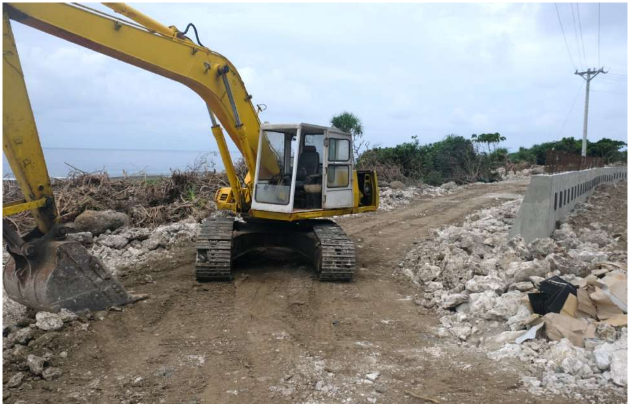
Figure 29 “Road Digger.” Concrete road expansion project under way. (photo by author)
