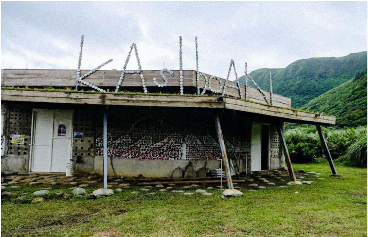
Figure 14 “Kasiboan.” This is event center and eco-activist hub is built from recycled PET bottles. (photo by author)
